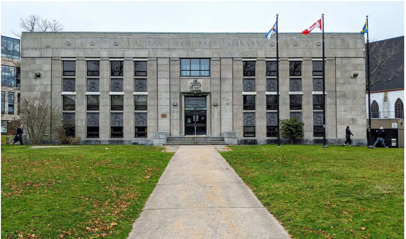
Front façade of the former Halifax Memorial Library and burial ground (courtesy of the author)
