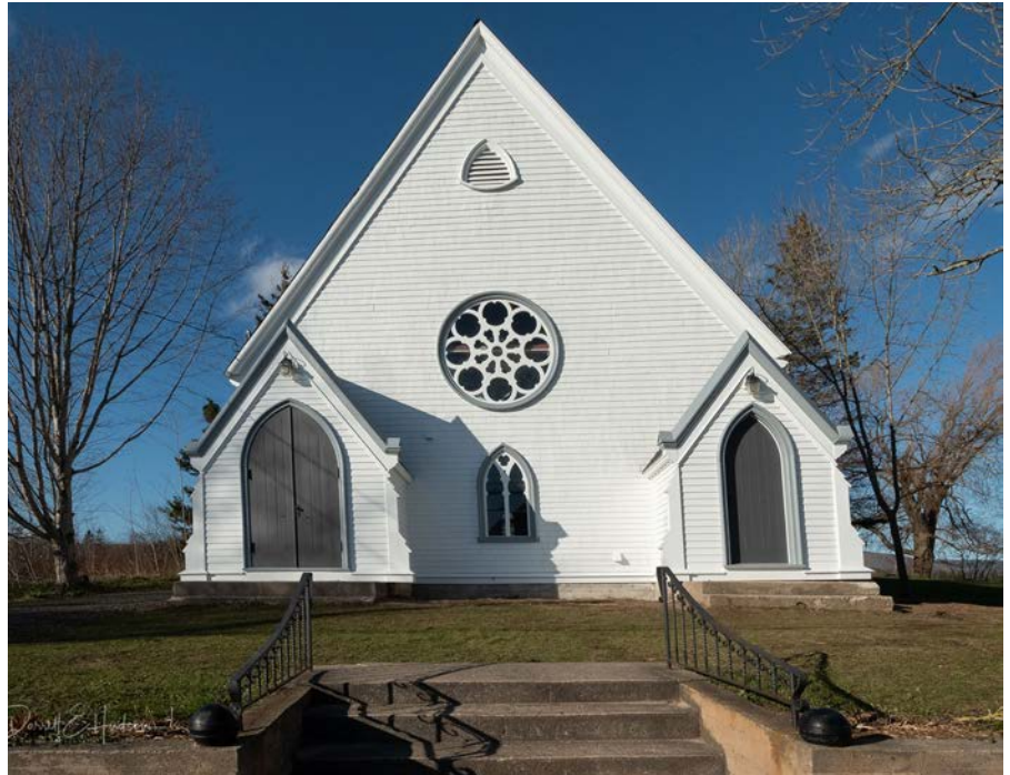
Dual entry doors and rose window, former Centenary United Church, Upper Granville (photo courtesy of Darrell Hudson)
