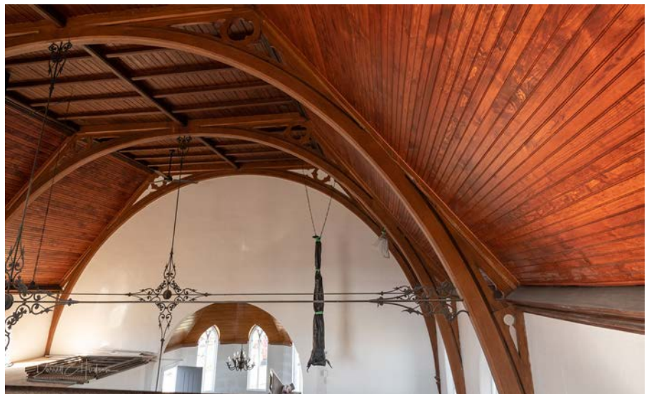
Roof structure and ceiling (photo courtesy of Darrell Hudson)
