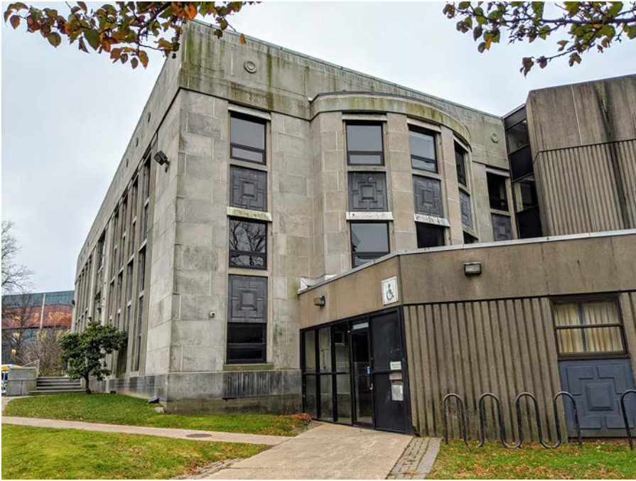
Former Halifax Memorial Library, showing part of 1970s extension, with a glimpse of the new Central Library in the background (courtesy of the author)
