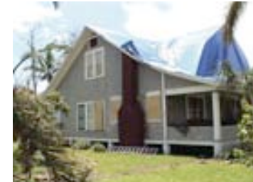
A roof tarp provides temporary stabilization.
