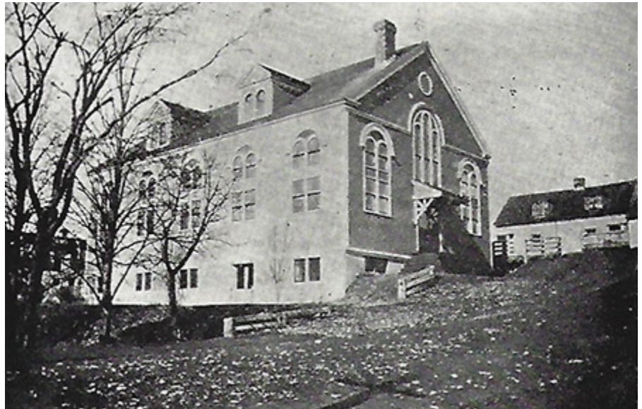
The present parish hall, as built, looking up Dundas Street to the corner of North; note five bays and large dormers, no longer present (courtesy Christ Church Historical Committee)
