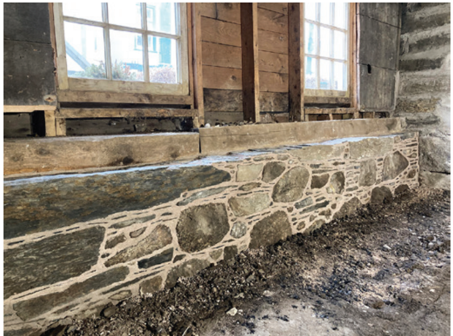
Repaired foundation wall (courtesy Lunenburg Heritage Society)
