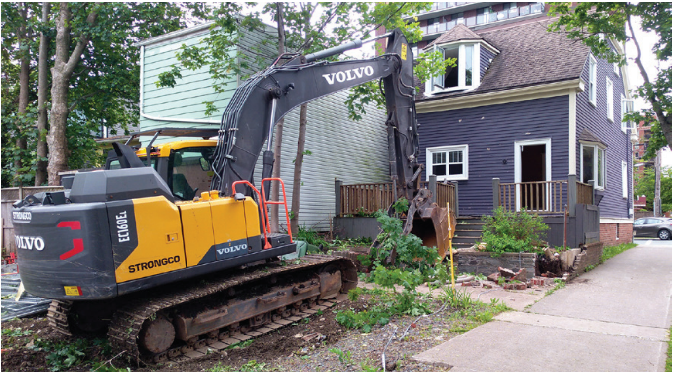
Heavy equipment poised to demolish 1195 Tower Road on 19 June 2023 (Griffin photo)
