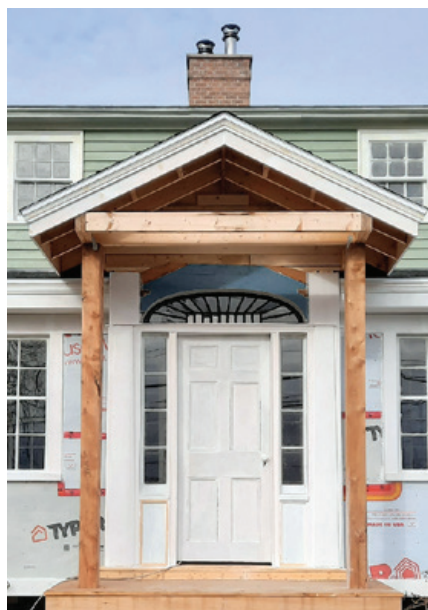
Salvaged door installed (author photo)
