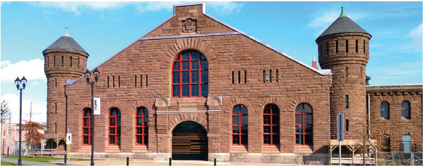
Rehabilitated west façade as seen from the Halifax Common (Griffin photo)
