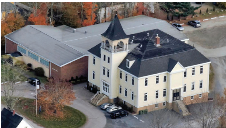
Aerial view of the Mahone Bay Centre, showing both parts of the building (courtesy of the author)
