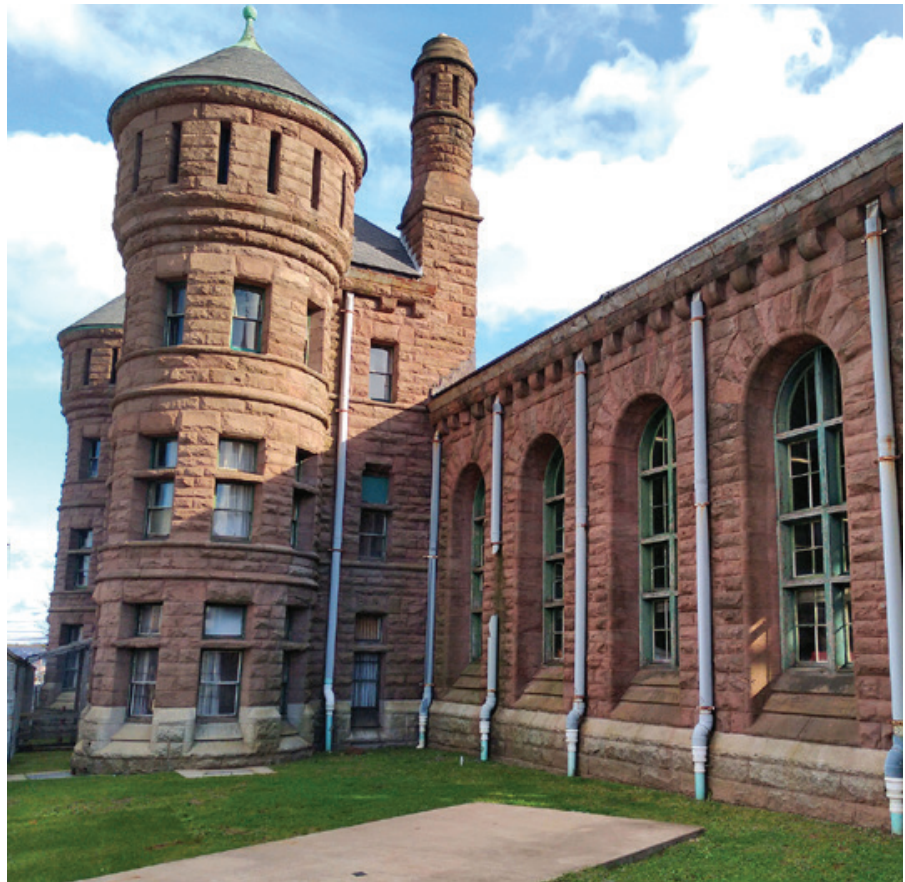
Row of windows lighting the drill hall and the ‘castle’ in the middle of the north façade (Griffin photo)
