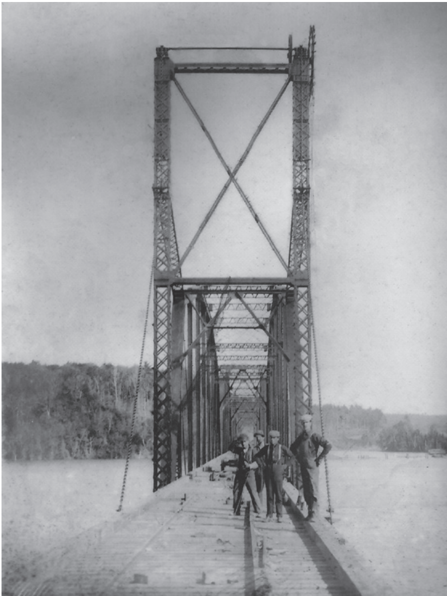
Workers laying rail on completed bridge (photo courtesy CHArt Society, Maitland)
