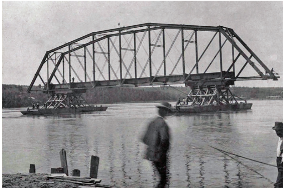
Floating span into place (photo courtesy of Jeff Yuill)
