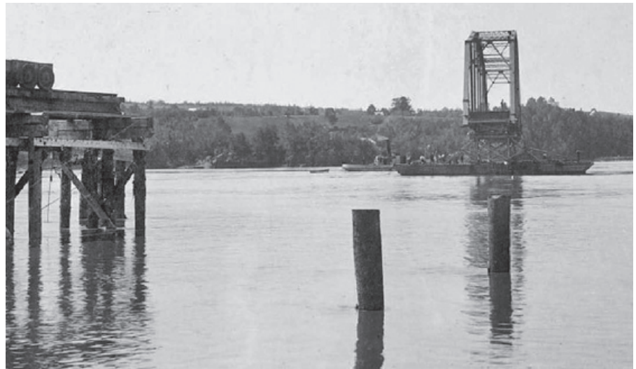
Span emplacement, showing scow and tug Bessie, viewed from west abutment (photo courtesy of Jeff Yuill)
