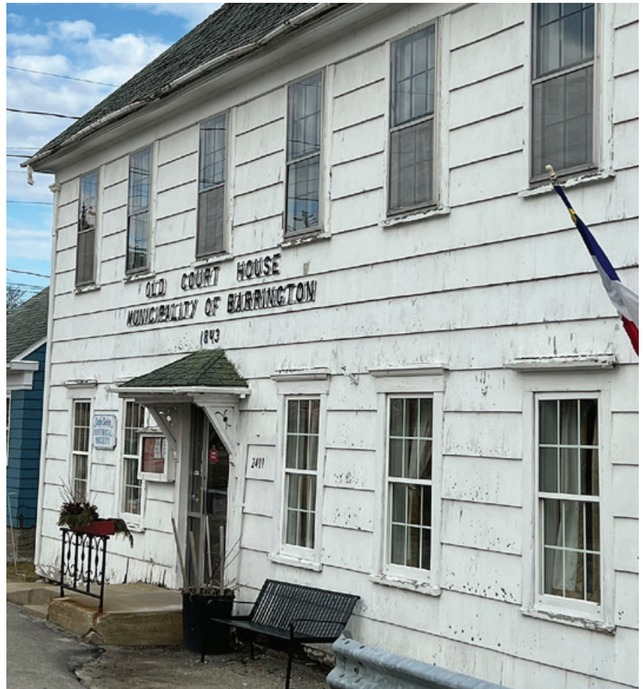
Façade and entry, Old Court House, Barrington (courtesy of Samantha Brannen, Director, Barrington Museum Complex, and the Cape Sable Historical Society)
