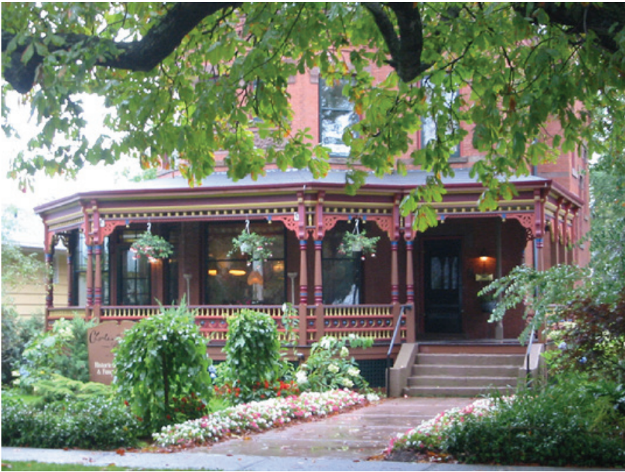
Charles Richards House, Yarmouth, front veranda (photo: D.L. Forbes, September 2005)
