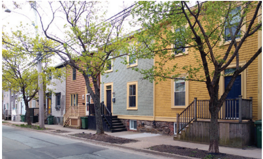
The last eight houses built by Henry J. Harris, 2344-2368 Maynard Street, seen from the north end (Griffin photo, May 2022)
