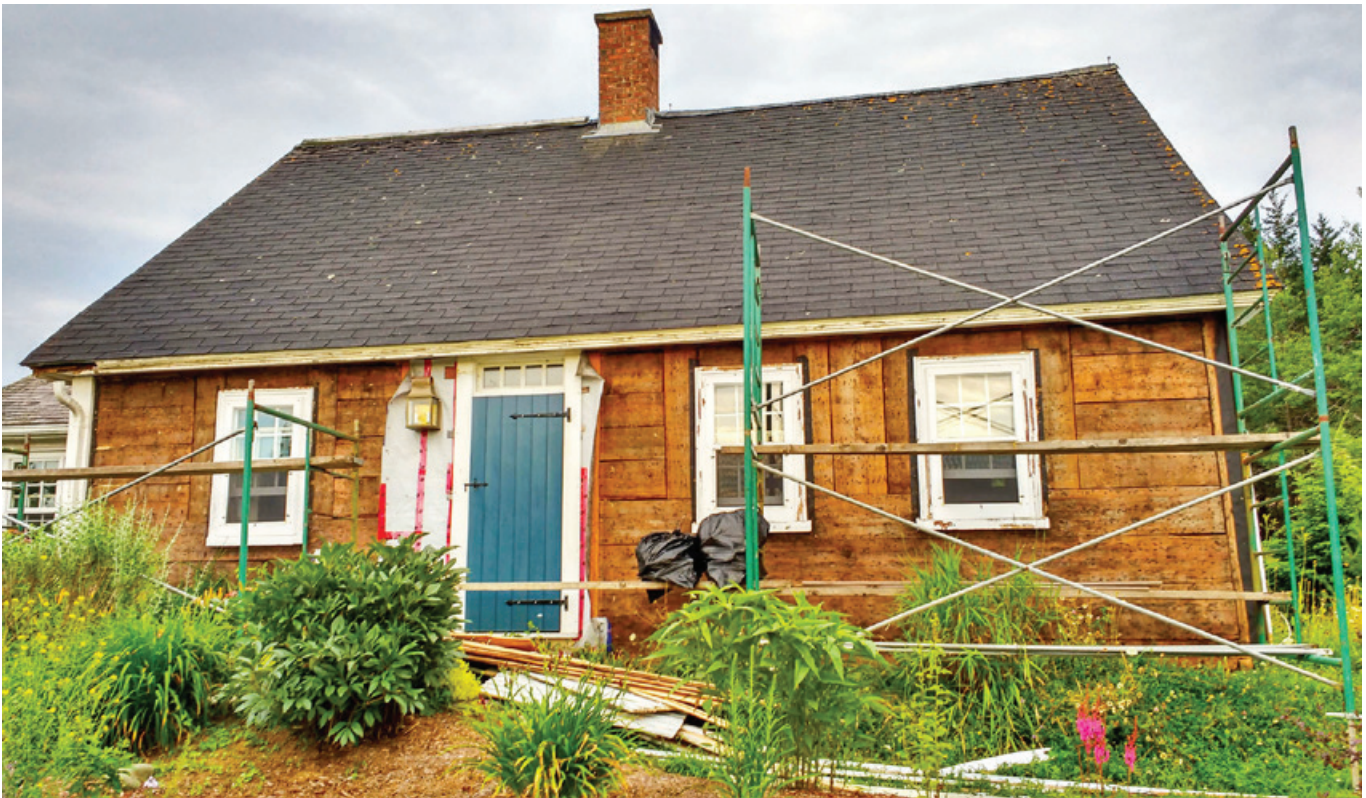
House façade laid bare, displaying coulisse framing (courtesy of the author)
