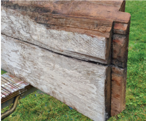
Coulisse wall board with tenon (left) and stacked and inserted into corner post (right) (courtesy of the author)
