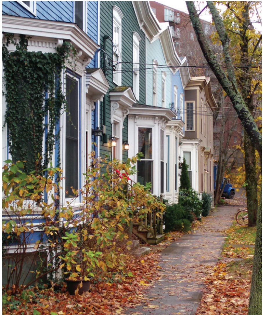
Another view of the rebuilt end of the Smith Street terrace houses (Griffin photo)
