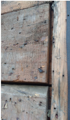
Coulisse wall board with tenon (left) and stacked and inserted into corner post (right) (courtesy of the author)
