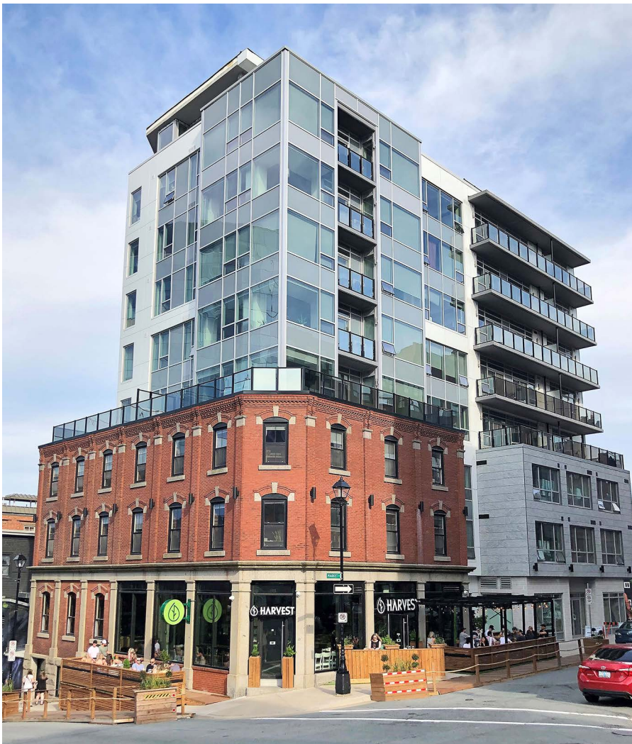
Redevelopment and densification retaining part of the historical building on the corner of Market and Sackville streets in Halifax
