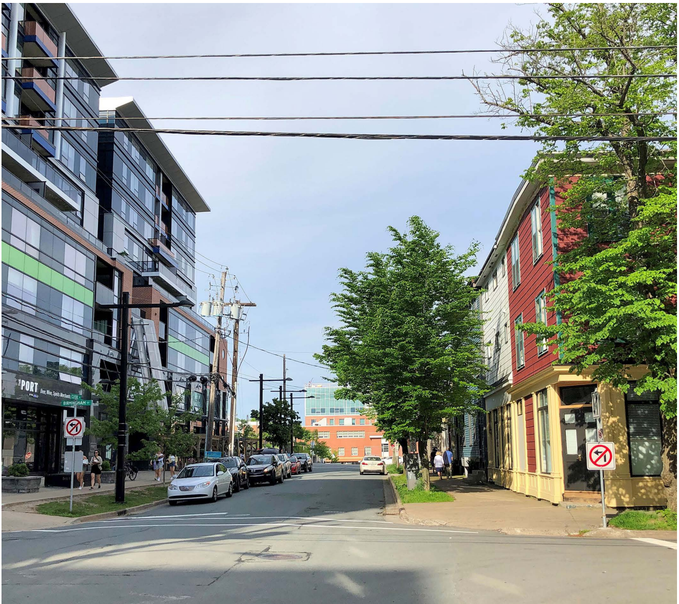
Many new developments such as this example (left) on Clyde Street do not fit the context of the surrounding neighbourhood, in contrast to scale-appropriate and sympathetic repurposing (building at right) featured in the December 2020 issue of The Griffin (v.45, no 4)
