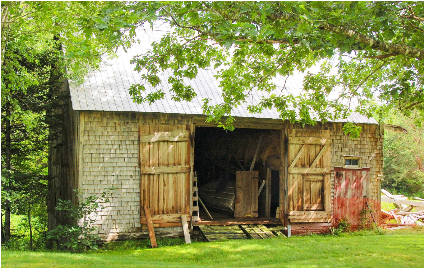
John Cruickshank's three-bay English barn, probably built in the early 1830s, in Caledonia, Guysborough County (photo by Meghann Jack)
