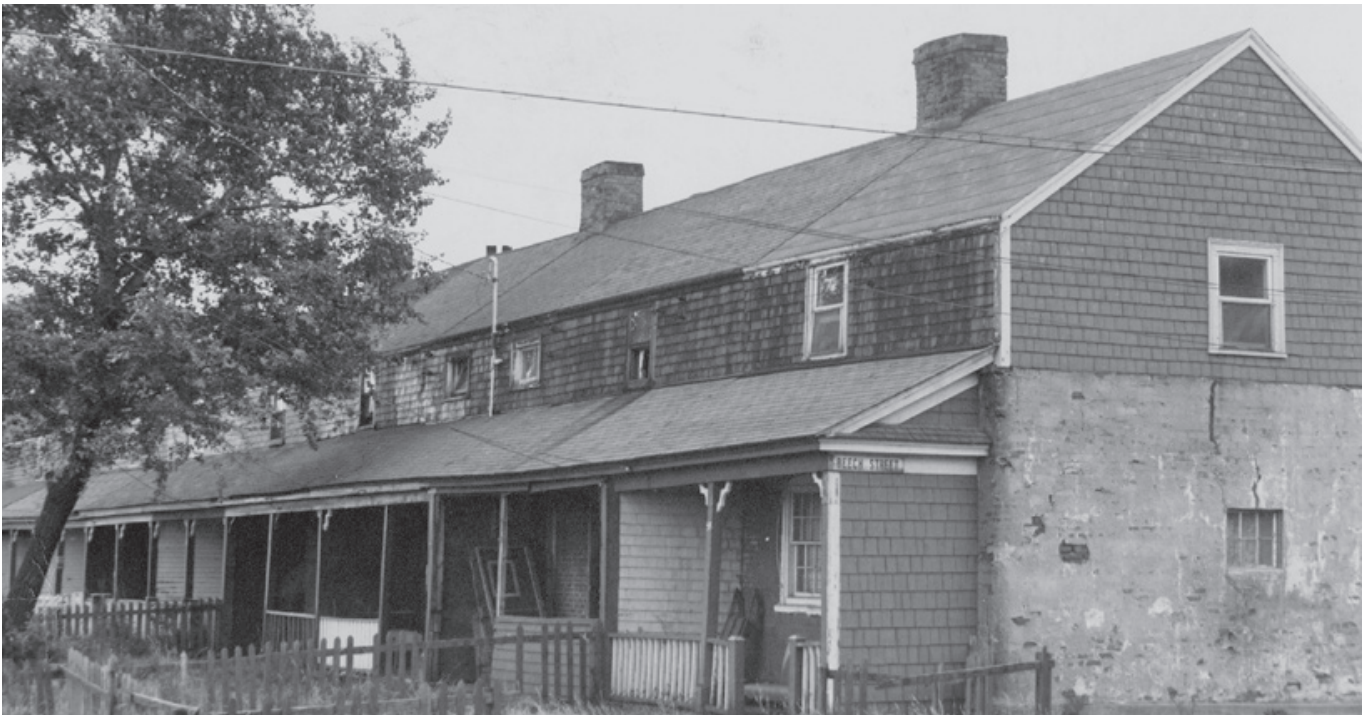
Red Row, showing post-1902 addition of upper frame full-storey (undated photo, c. 1970s, Museum of Industry, 191645 GMA SM003)
