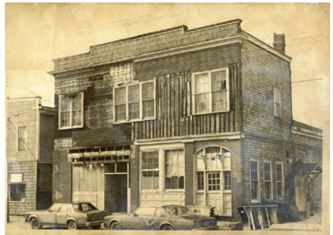
Former King's Theatre having fallen into disrepair, 1981
