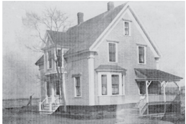
Older photo of the home (courtesy Annapolis Heritage Society)
