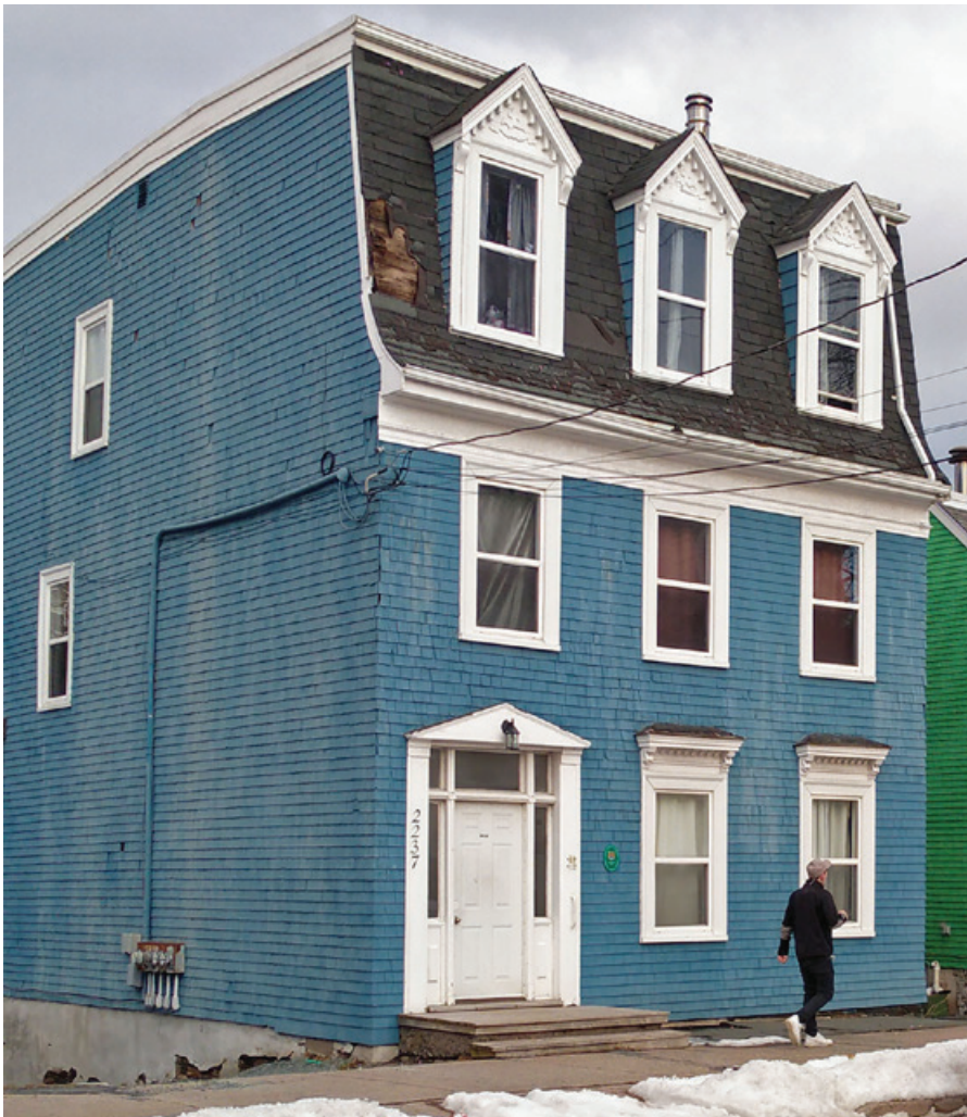
The Smyth House today, without the storm porch, February 2021 (Griffin photo)
