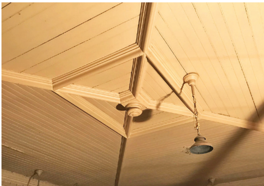
Preserved ceiling uncovered in former corner store
