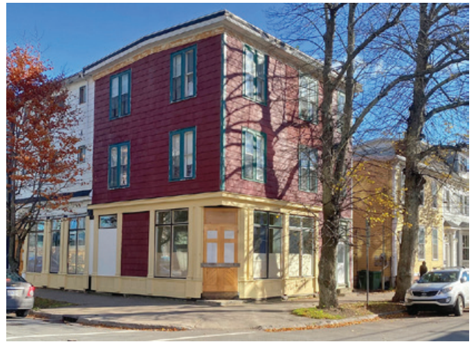
The building as it appears today (Clyde Street to the left, Birmingham to the right)
