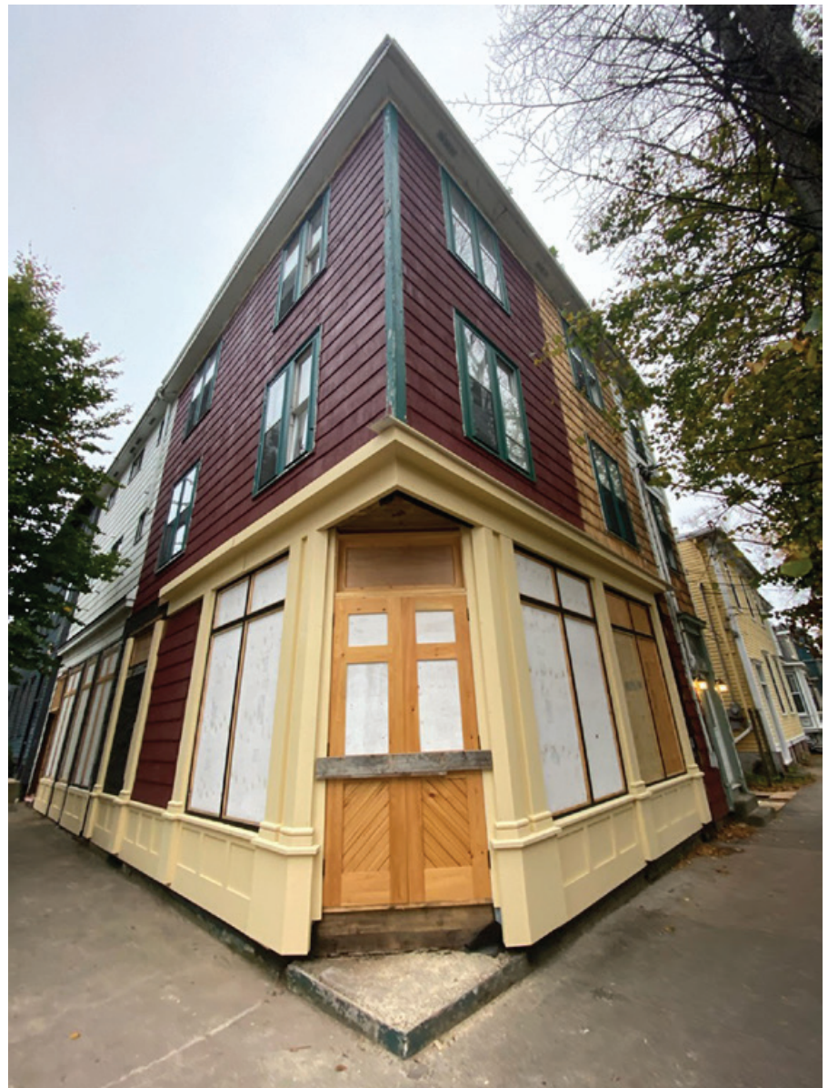
Restored shop front at the corner of Birmingham and Clyde streets, Halifax (accessible entrance at far right end of building)
