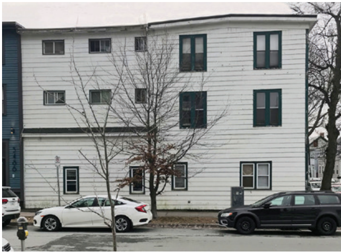
Former stores (corner and liquor), Clyde Street elevation, before work began
