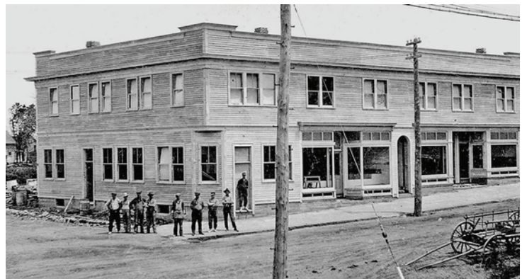
The newly completed Cummings Block, 1922 (courtesy of the Annapolis Heritage Society)
