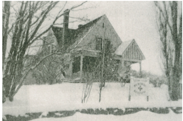
The Fraser house as a Red Cross Outpost Hospital (courtesy Northumberland Arts Council)
