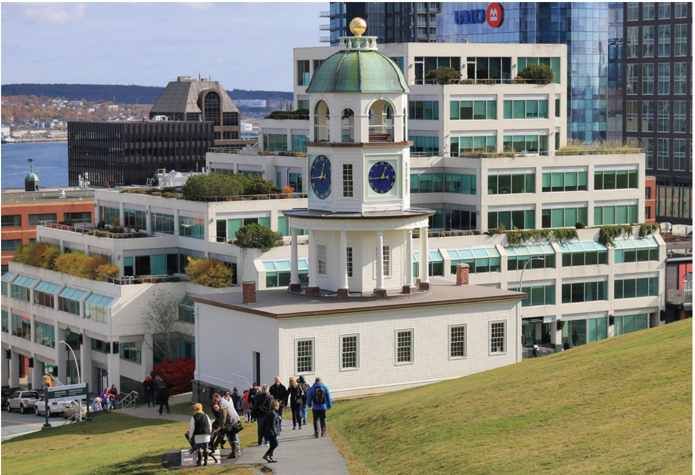
The project completed, October 2019; despite new curtain walls and rising roof lines, the harbour can still be glimpsed (note St Paul's Church cupola peeking above the roof of the Prince George Hotel)
