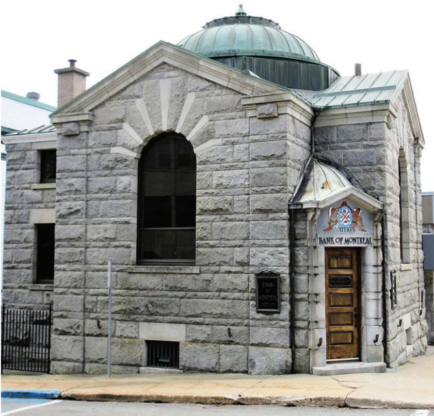
Finished project with restored corner doorway
