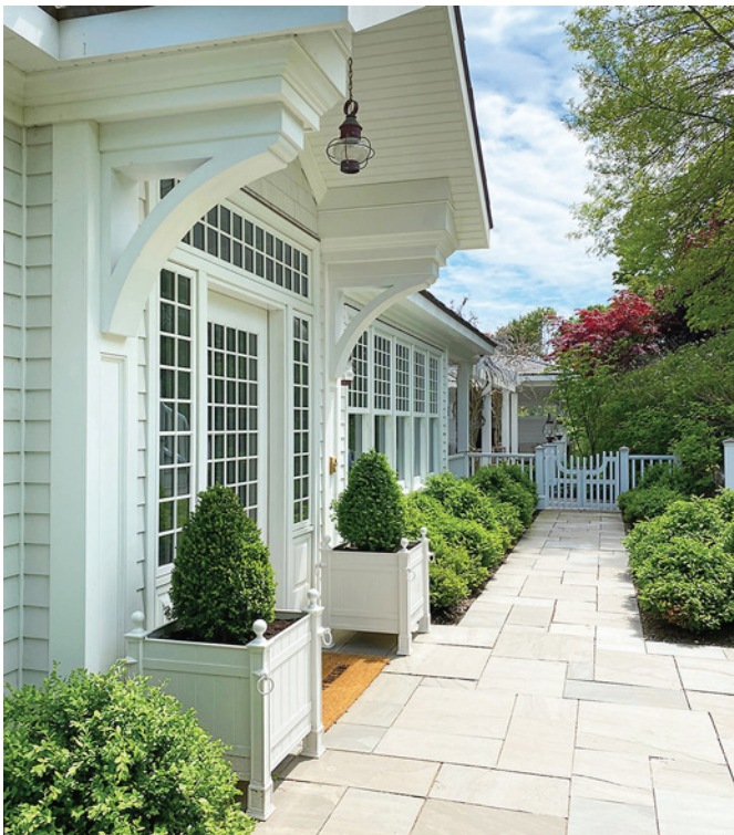
Front entry, exterior and interior, after restoration
