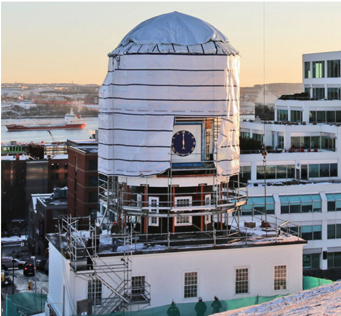
Scaffolding was erected over the entire turret, including the ball, December 2018 – a strange-looking tower overlooks the city's historic precinct and harbour
