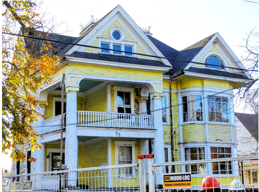
John Alfred Laws House (1907), 23 Spring Street, Amherst (photo courtesy of Lisa Davison)
