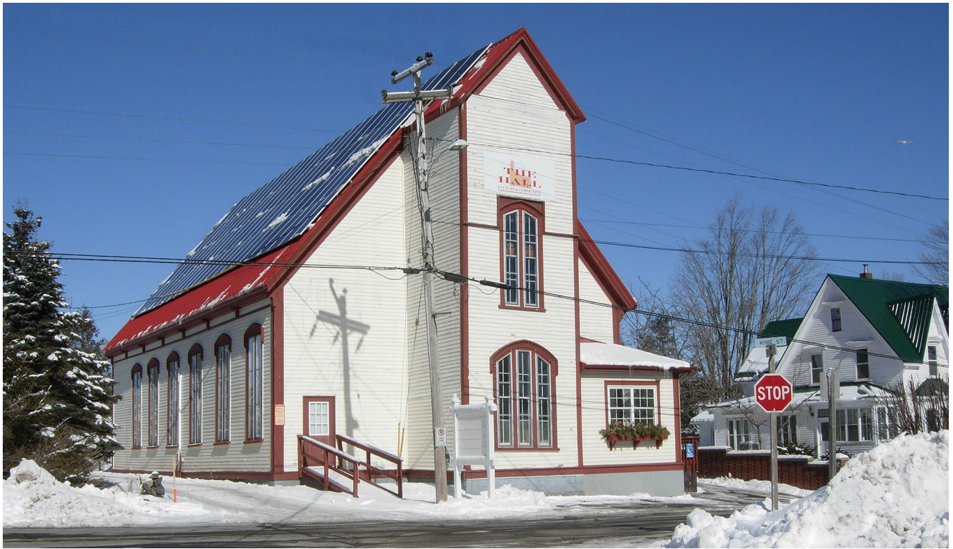
The Hall as it looks today, with truncated tower, new roof, solar panels, and near-original window trim (courtesy Janet Doble)
