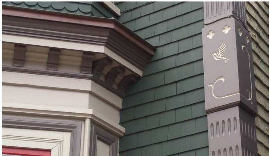
Detail of bay, corner boards, and new carving incorporated in corner board to mark the restoration project (Griffin photo)
