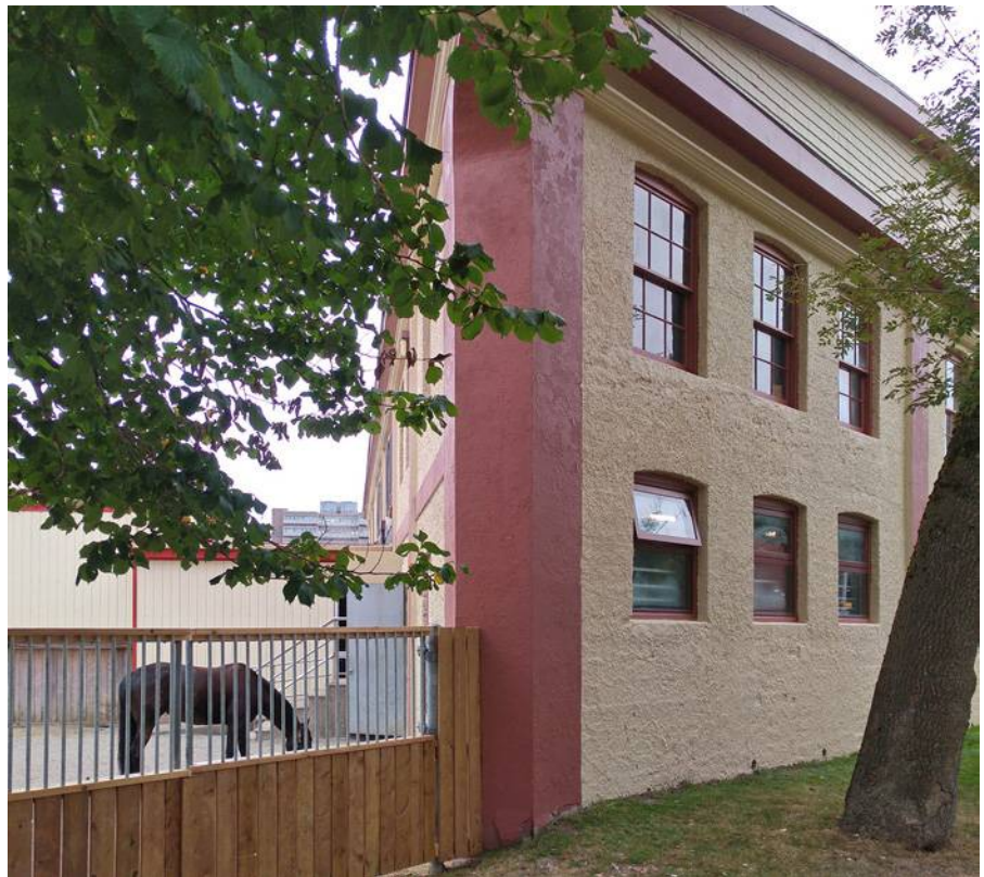
Halifax Lancers' stable, Bell Road façade with 'pointed' corner (Griffin photo)
