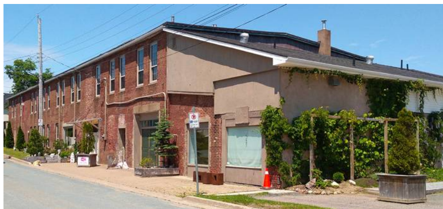
The Cedar Centre, Windsor, venue for the 2019 Heritage Trust awards ceremony and winner of the 2018 award for conservation and adaptive re-use of a heritage industrial building (Griffin photo)
