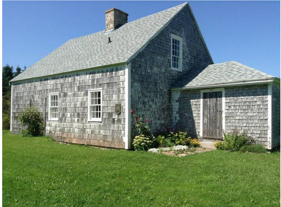
Exterior view showing 6-over-6 and 9-over-6 windows, central chimney and provincial heritage plaque (courtesy of Diana Pereira)
