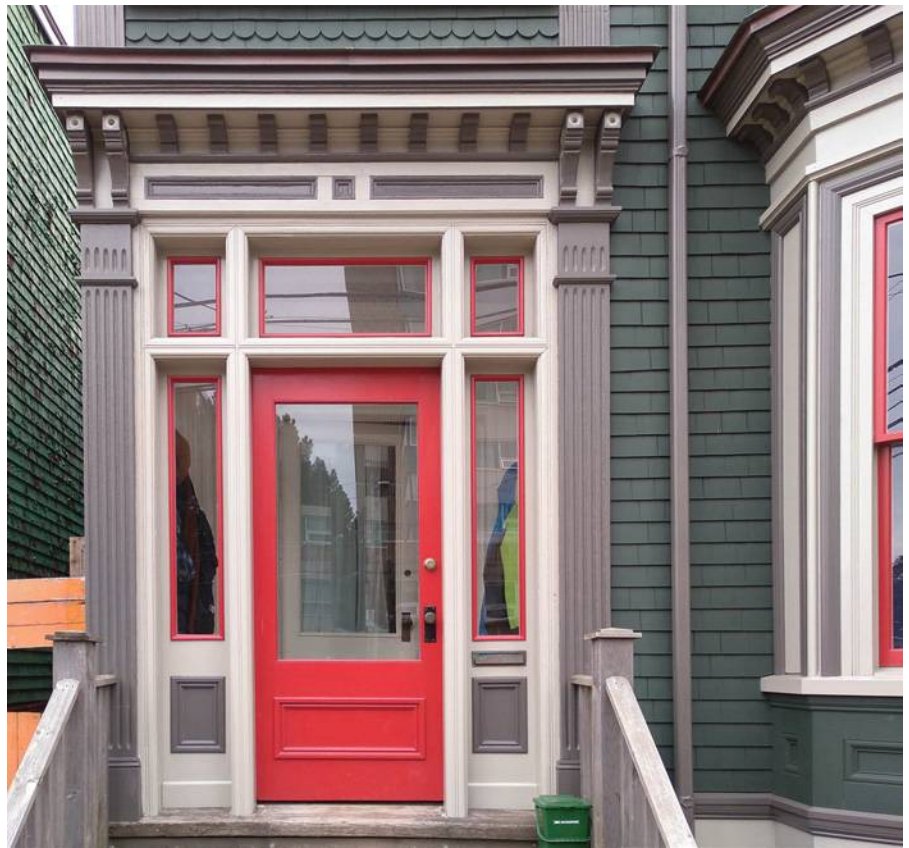
Front entry, 5518 North Street (Griffin photo)
