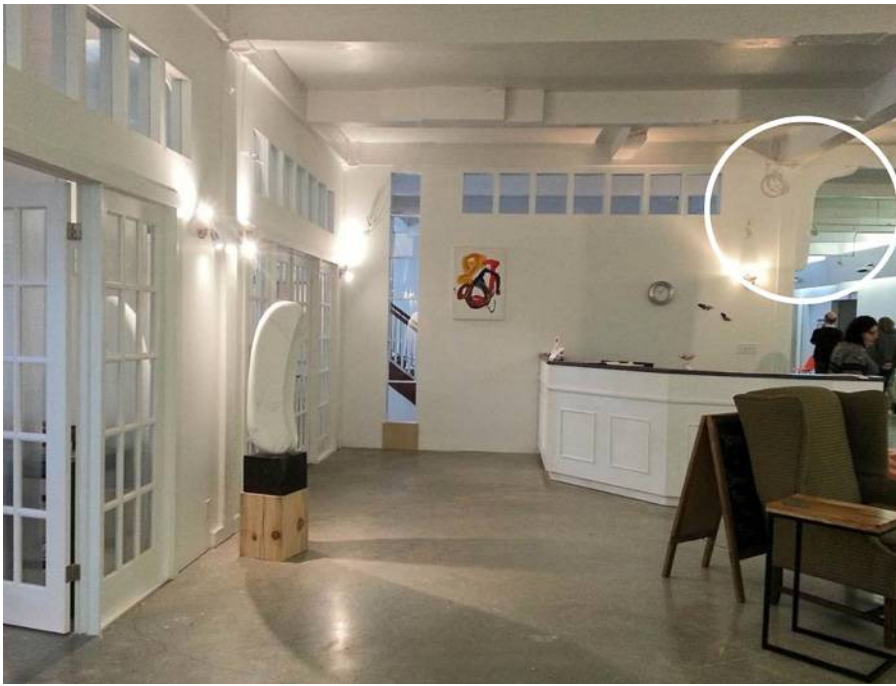
Reception area with multiple French doors and transoms allowing light into the lower interior space; main staircase visible in the background through vertical window; large timber knee (circled) can be seen at far right (photo courtesy of the Cedar Centre)
