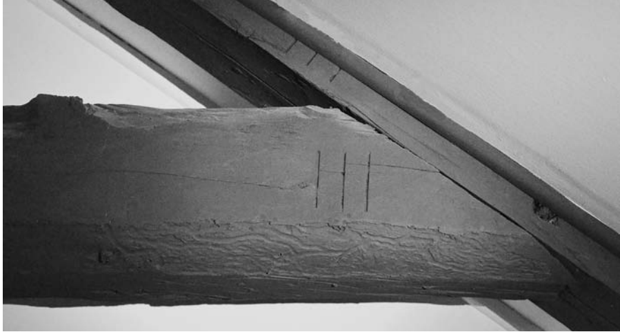
Roman numerals in third-storey timbers (Griffin photo)
