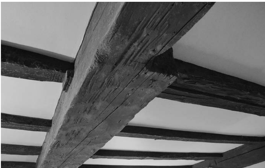
Notch for central chimney in ceiling beam (Griffin photo)
