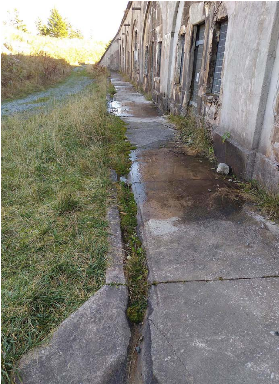
Carved stone pavement and drain along row of casemates, Fort McNab, November 2018 (Griffin photo)
