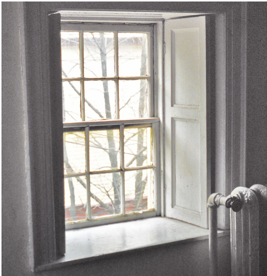
Panelled window recess in upstairs bedroom of the original cottage; radiator added later (courtesy of the author)
