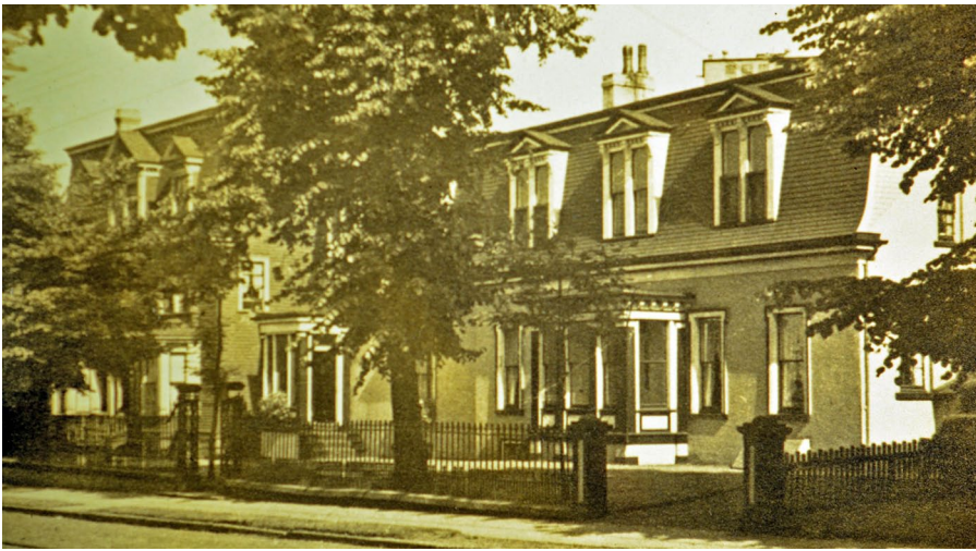
The house circa 1930, showing the three dormers in the mansard roof and the iron fence dated 1832 (courtesy Frieda Chipman)
