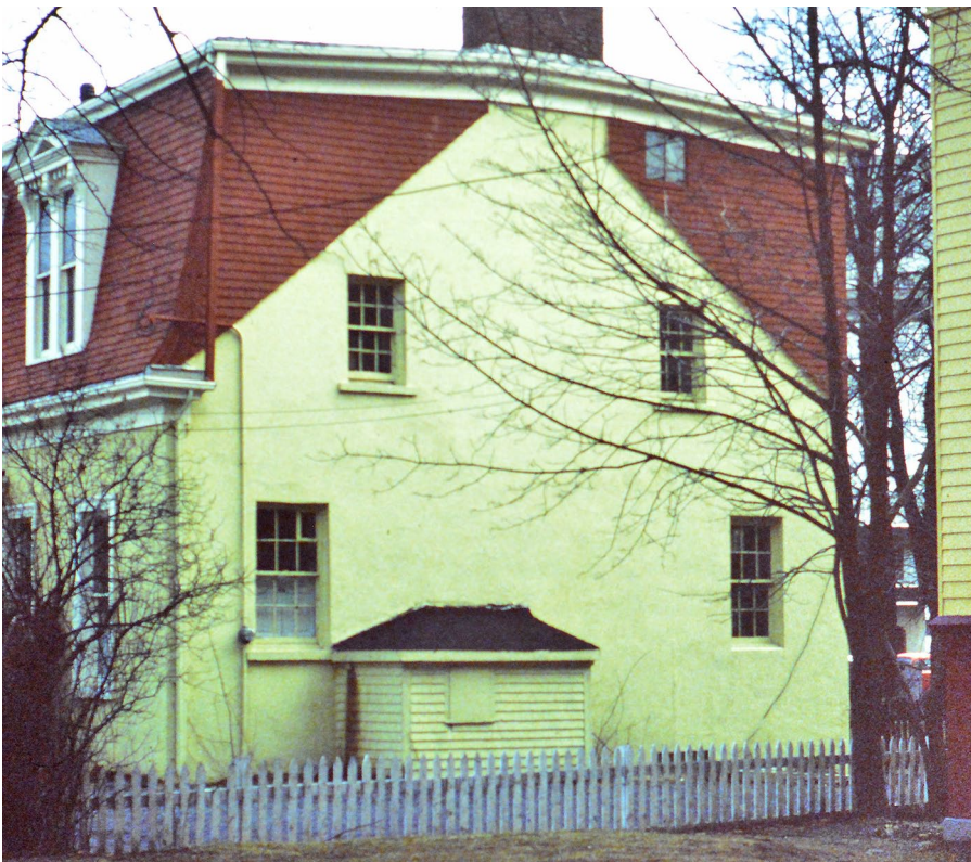
Gable-end view of the house in 1979, showing original roof line (as seen in the Mercer painting) with Victorian mansard superimposed (courtesy of the author)
