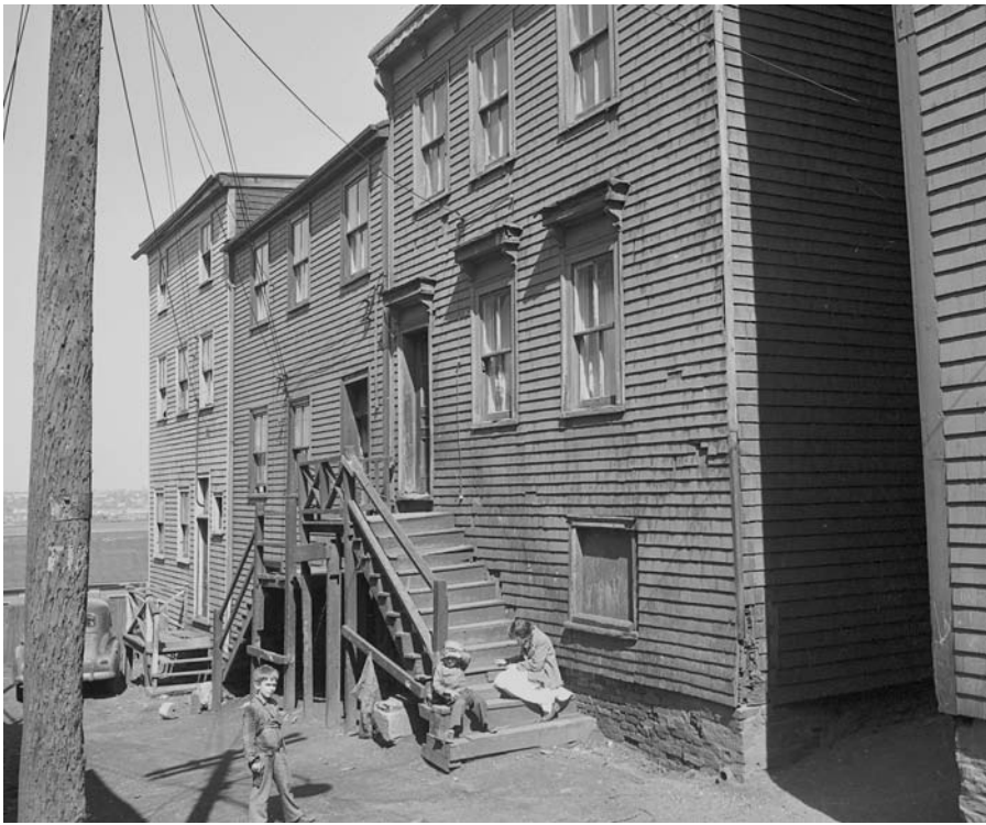
Elevator Court, late 1950s or early 1960s (Halifax Works Department photograph, HMA, 102-39-1-1401.14)
