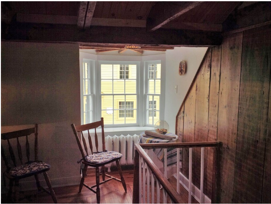
Upper landing with view through front dormer and exposed cladding of the 'house-within-a-house' (Griffin photo)
