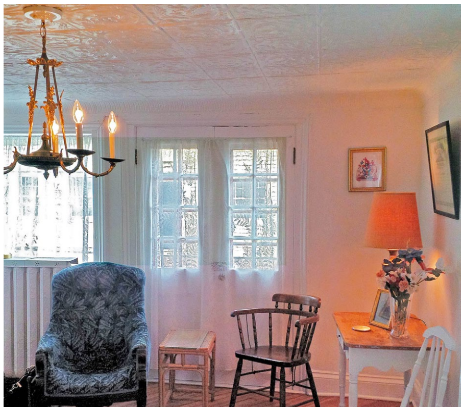
The house has tin ceilings in the former Customs office (seen here) and other parts of the main and lower floors; note double doors opening to the street, as seen in the historic photo (Griffin photo)
