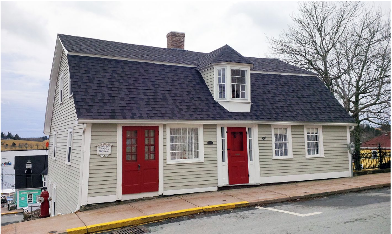
Pelham Street façade of the Ältestes Haus (Oldest House) in Lunenburg; note harbour view, Duke Street at left, side lot at right, plaque, and hydrant at the corner (Griffin photo)
