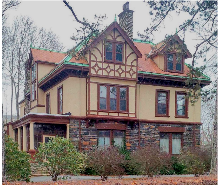
Ardnamara, 851 Young Avenue, before demolition (courtesy of Barry Copp)
