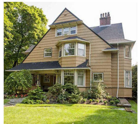
G.S. Campbell House, 825 Young Avenue, before demolition (courtesy Barry Copp)
