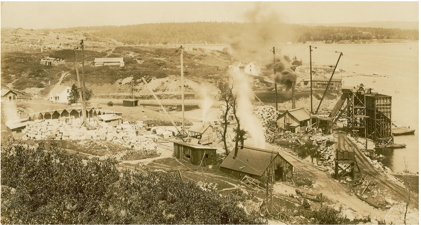
Overview of cutting shed, crushing plant, and wharf, with two homes and bare rock on hill beyond, 17 July 1916 (Gauvin and Gentzell, J.P. Porter no. F82, courtesy of Nova Scotia Archives)
