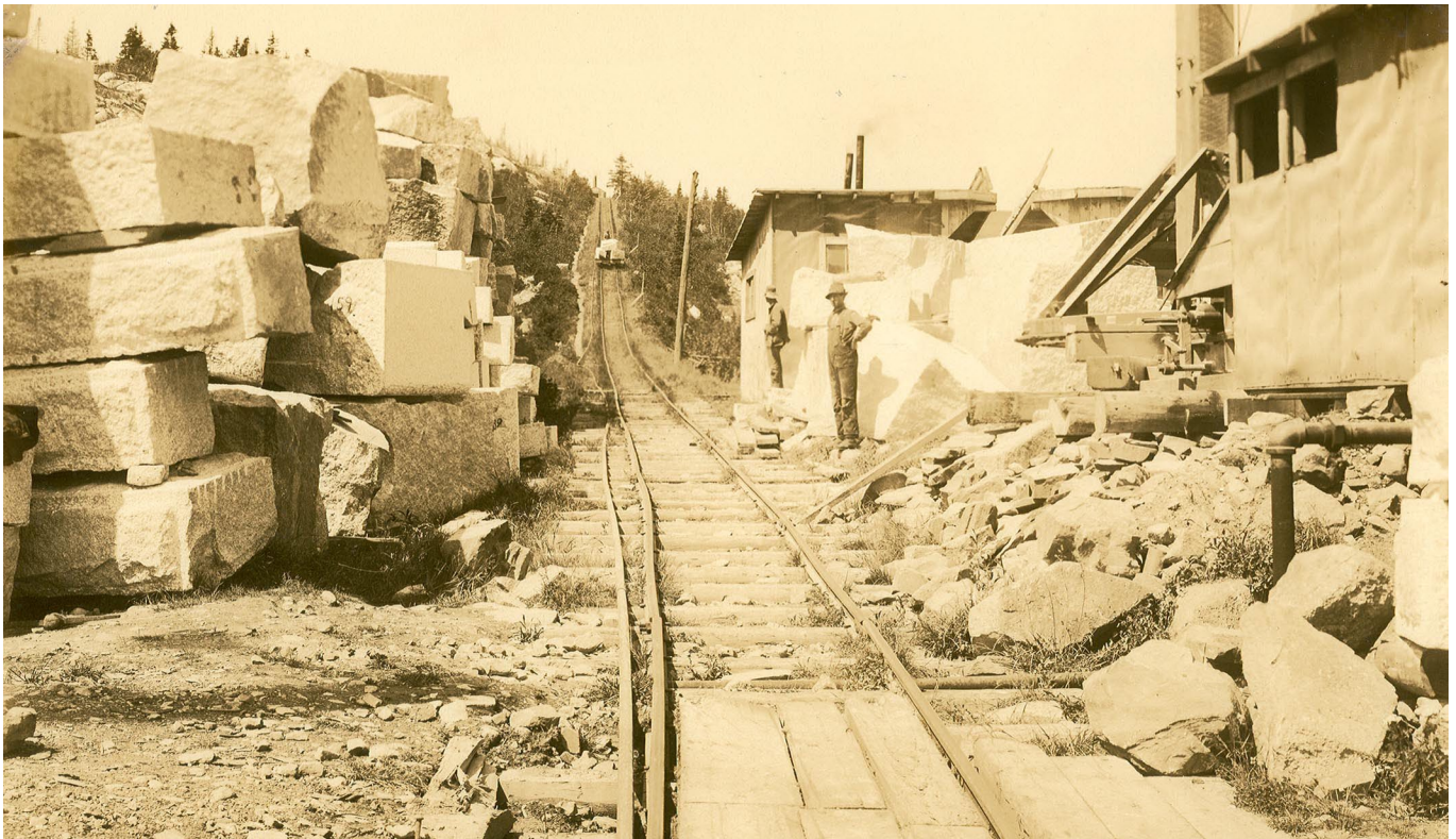
Tramway for cut granite at Purcell's Cove, 17 July 1916 (Gauvin and Gentzell, Foley Brothers no. F84, courtesy of Nova Scotia Archives)
