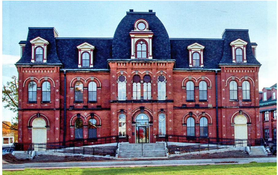
Restored exterior façade of the Normal College building in its new role as the Colchester East Hants Public Library, November 2016
