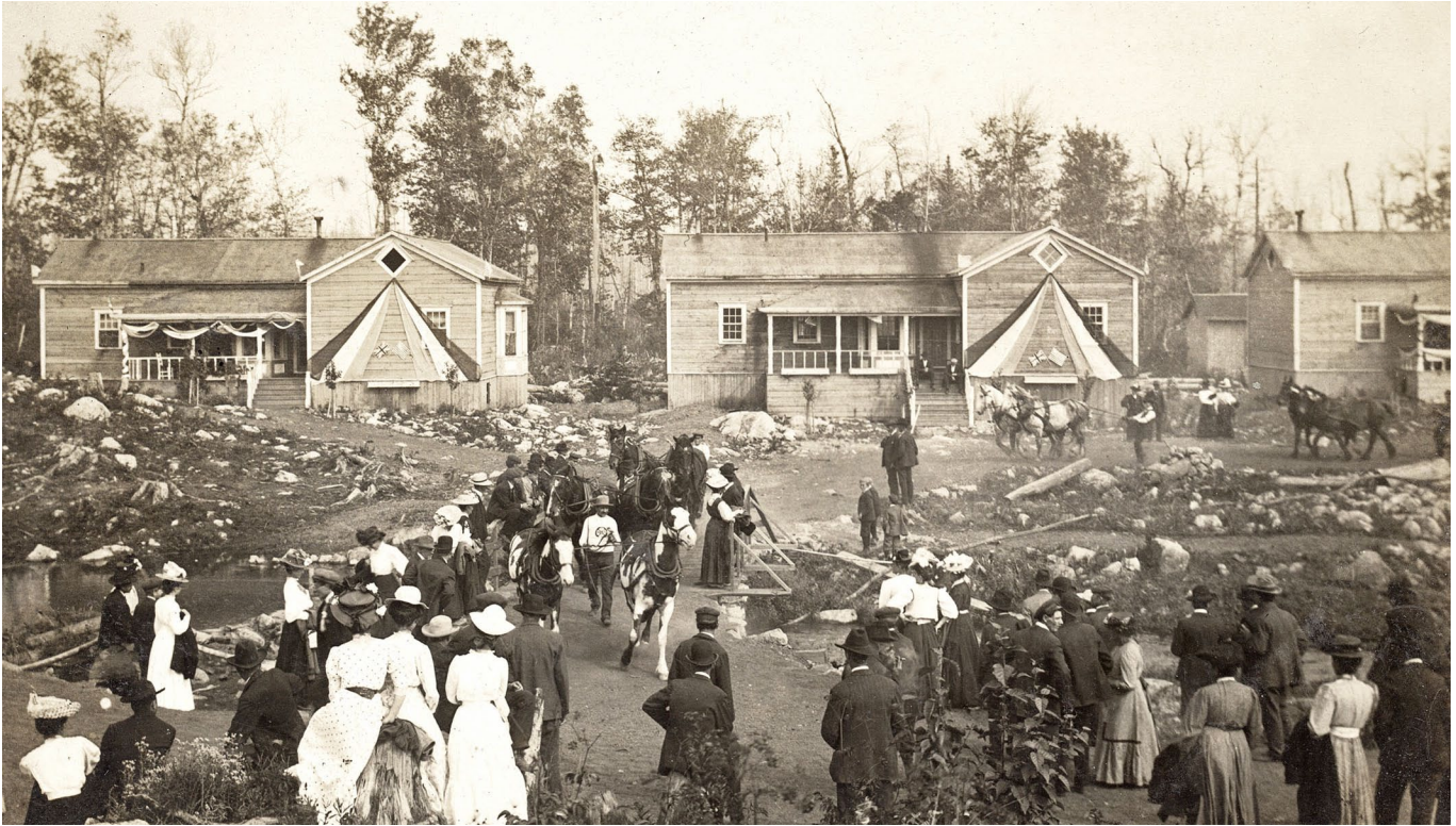
Fair day in Crossburn, with managers' houses in the background (note verandas and bay windows), bridge over stream, teams of horses; postmark on card is 1909 (courtesy of the author)
