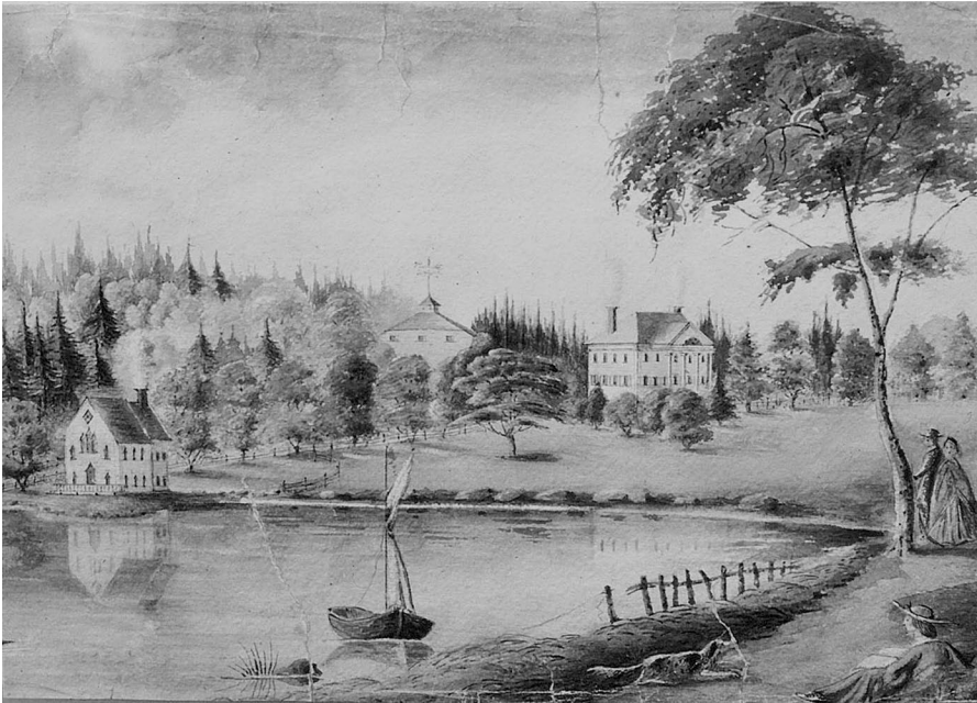
The core of the estate looking north, based on a similar view by Woolford: the male guest house can be seen in the lower left beside the lake; the Gothic Revival part nearest the water is obviously not a boathouse, and the two parts do not match (courtesy of the author)
