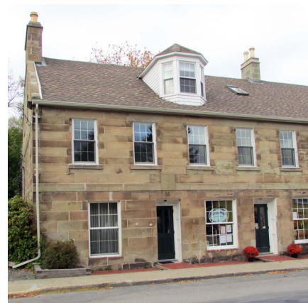
Street façade (courtesy Diane MacNeil)
