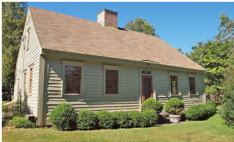
The original house built by Samuel Mack in Mill Village has all the characteristics of a mid 1700s New England dwelling (courtesy of the author)
