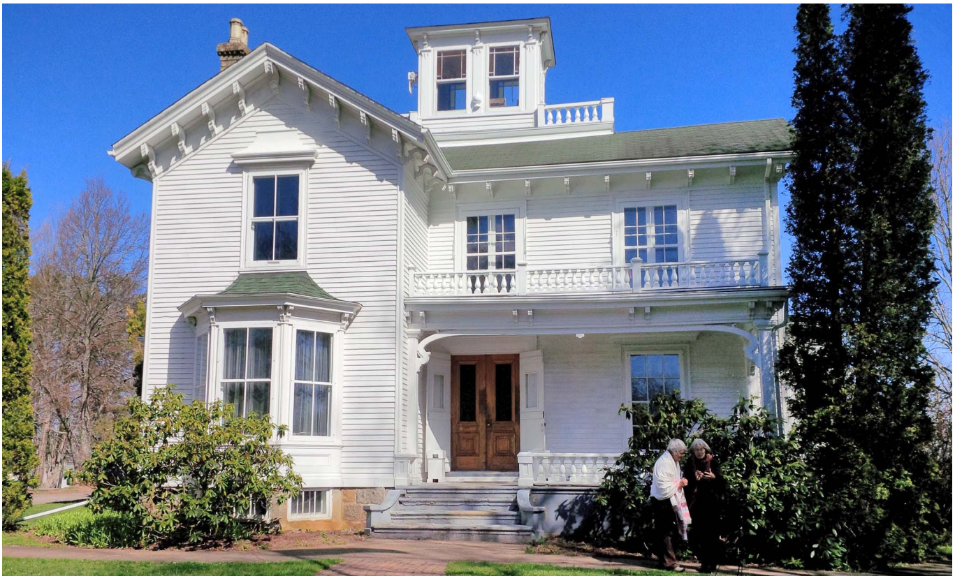
Front façade of The Cedars, showing bay, veranda, upper balcony, and widow's walk (Griffin photo)
