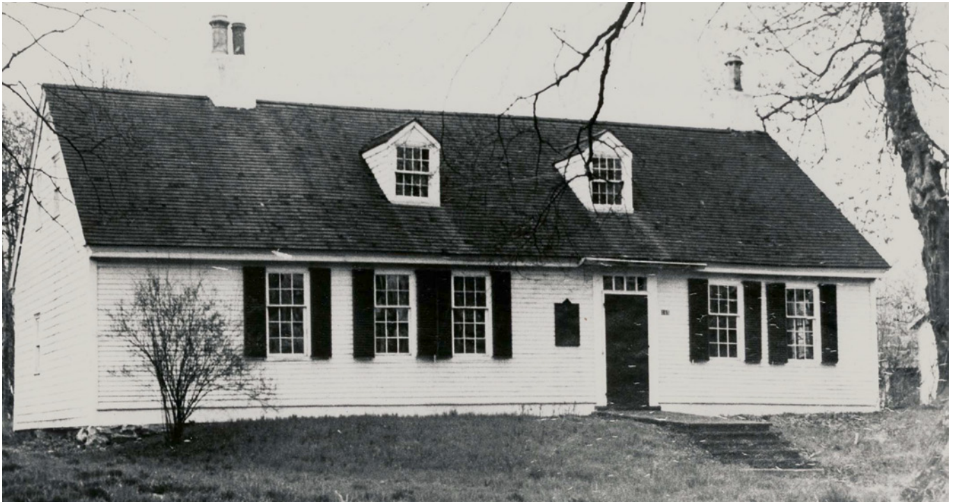
Simeon Perkins House, Liverpool, c.1950 – restoration work carried out in 1947 clearly left the building drooping over the partial cellar (author's photo of original in Queens County Museum)
