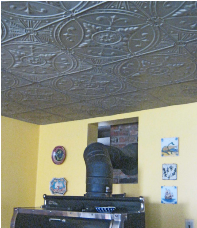
Embossed tin ceiling tiles rescued from a dump site by Willie; repaired, painted and installed over the wood stove in the kitchen (author photo)
