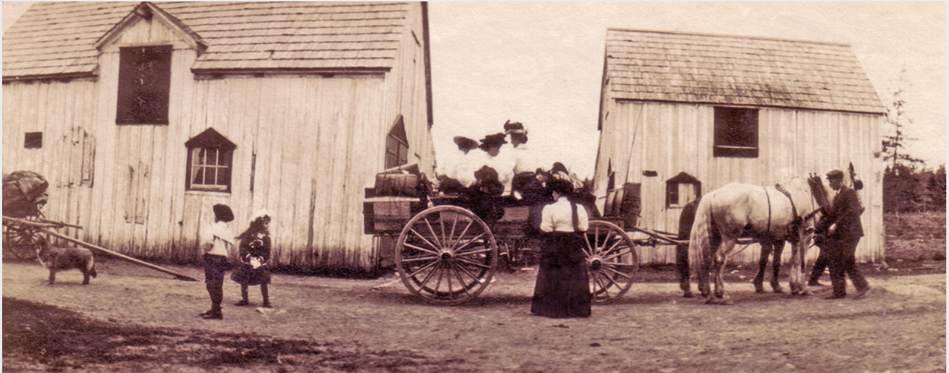
'Coach' preparing for departure at 14½ Mile Roadhouse (1912). This location is now on Parker Lane in Porters Lake. We see the barn (with a central dormer giving access the loft; the doors are open in the photo below) and a large shed; part of another vehicle is visible at left. Courtesy of Eastern Shore Archives (image D0079P051).
