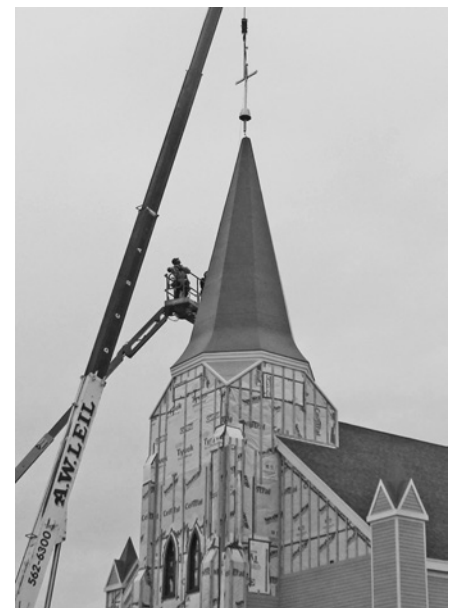
Raising the cross to top the new steeple on the rebuilt St Mary's Polish Church in Whitney Pier, 29 February 2016 (photo courtesy of Sajive Kocchar)
