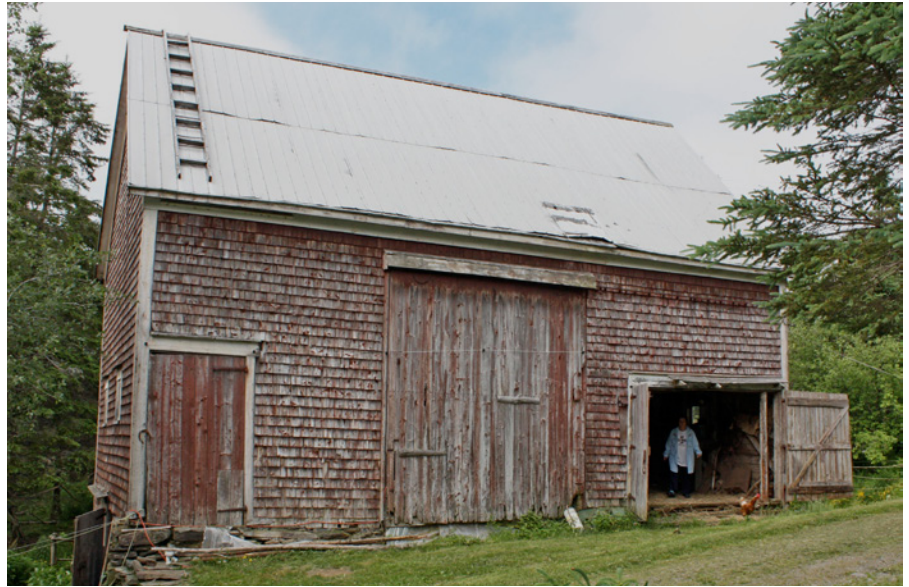
Typical three-bay English barn with centre-bay threshing floor, Moser River
