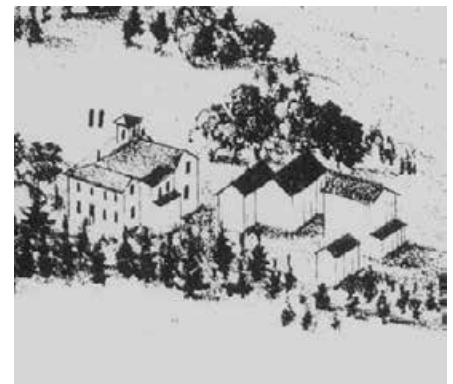
Clifton (1878) from Bird's Eye View lithograph, showing ancillary buildings (AP detail from original in Library and Archives Canada)
