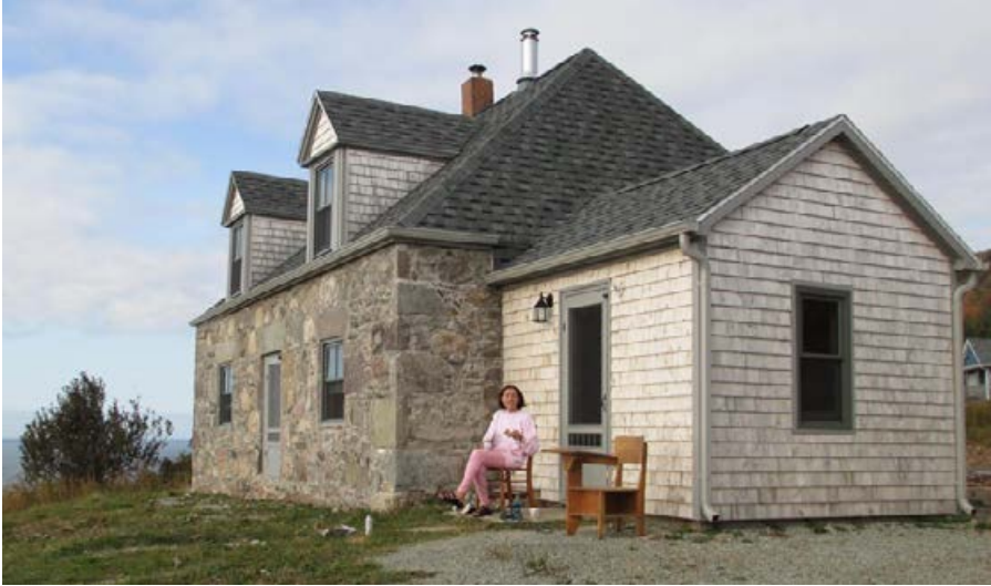
Enjoying the view, with exterior restoration completed (photo courtesy of the author)
