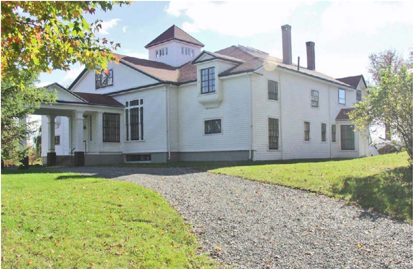
Post-1920 configuration, with porte cochere, high roof, and north porch added, the last major changes to the form (photo courtesy of the author)
