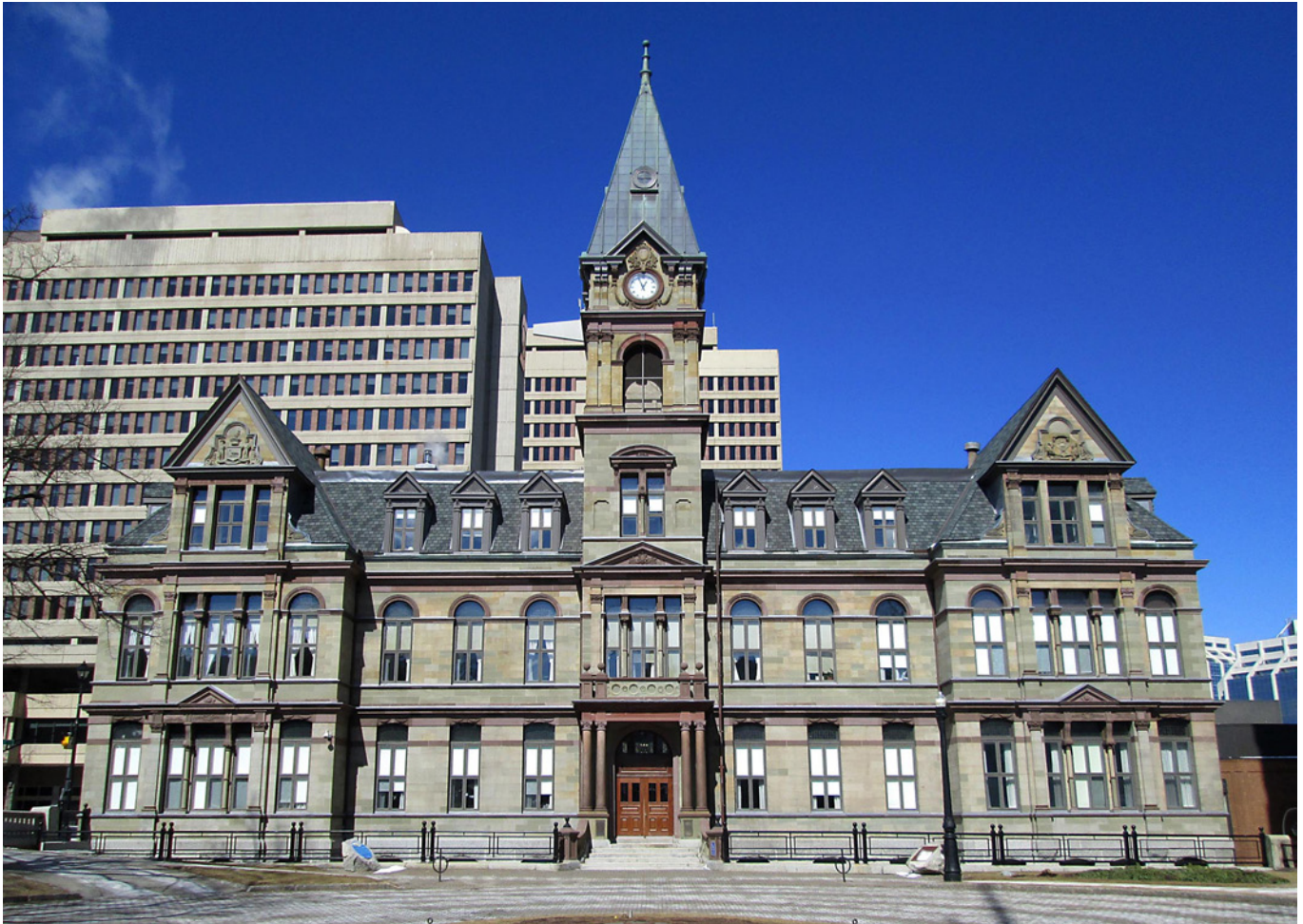
Halifax City Hall, venue for the February 2015 awards ceremony and recipient of award for the Masonry Conservation Program (photo courtesy of Halifax Regional Municipality)
