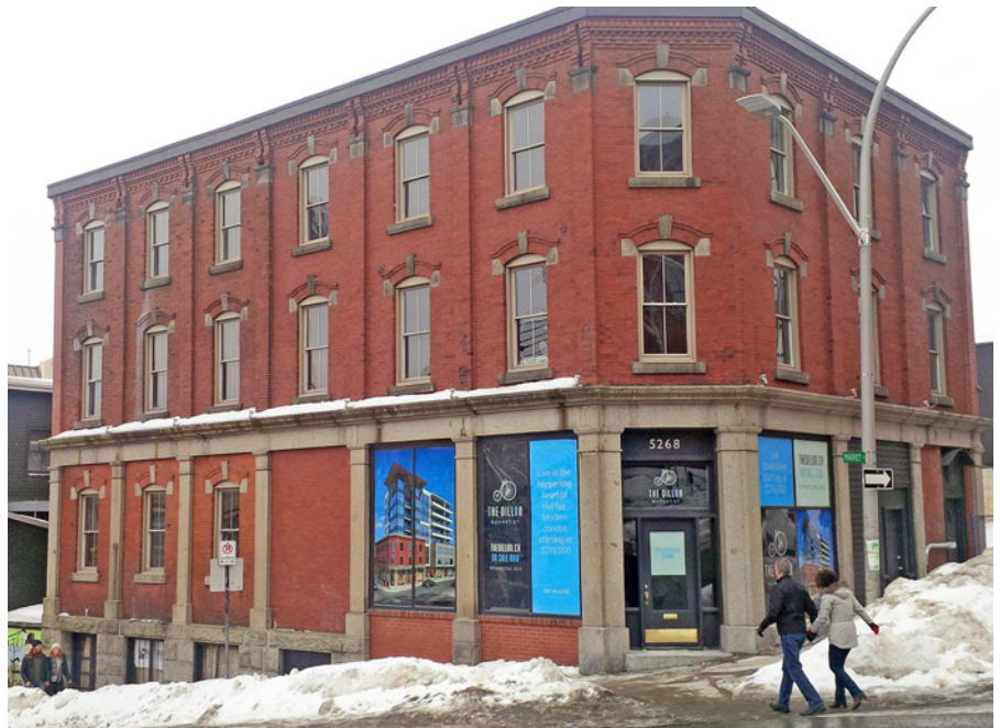
Dillon Building, with advertisement for new development, March 2015 (photo by Don Forbes)
