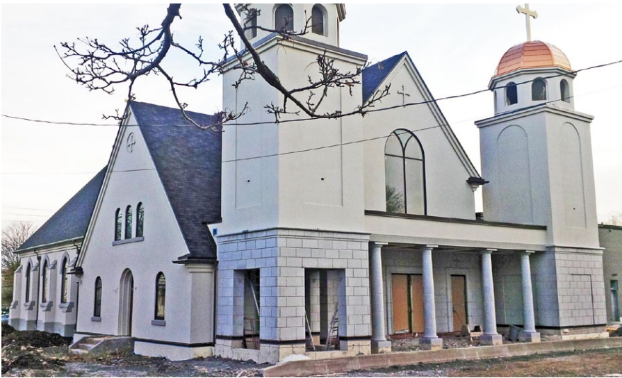
Nearly completed St Antonios Antiochian Orthodox Church, Halifax (former St Matthias Anglican Church) at the corner of Windsor Street and Chebucto Road (Griffin photo, November 2014)
