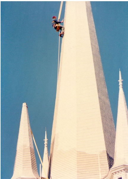
Steeple maintenance in 1979
