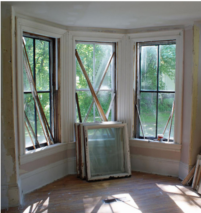
Renovations underway, interior of side bay
