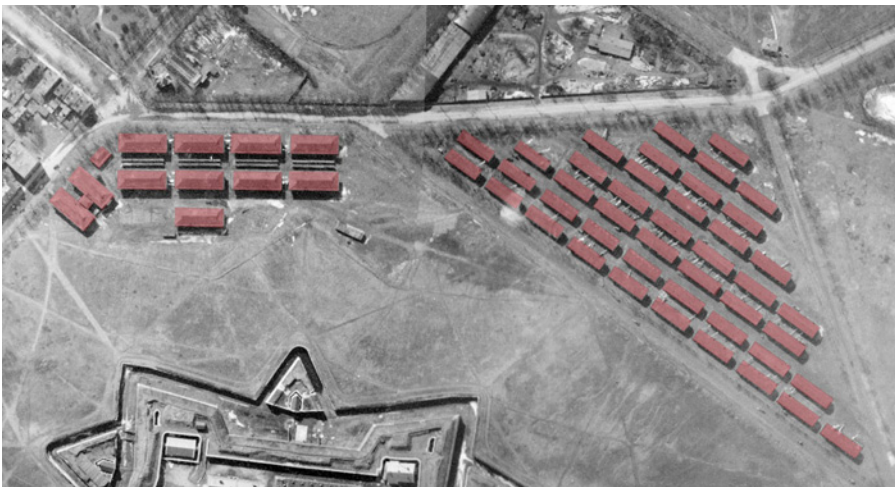
Building footprints in the area of the Garrison Grounds are highlighted on the air photos (1921 air photos courtesy of National Air Photo Library, Natural Resources Canada)
