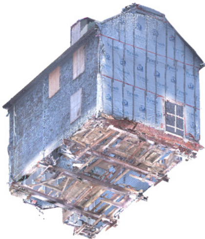
3D point-cloud model of the Morris House, acquired prior to the move in 2013, clockwise from top left: street façade (east wall) and south wall in new location; street façade and north wall in new location; underside, north wall, and back (west) wall in new location; underside as used to design new foundation (courtesy of the author)
