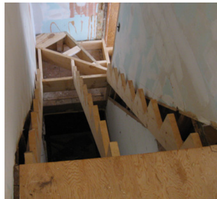
Main stair stringers and winder framing
