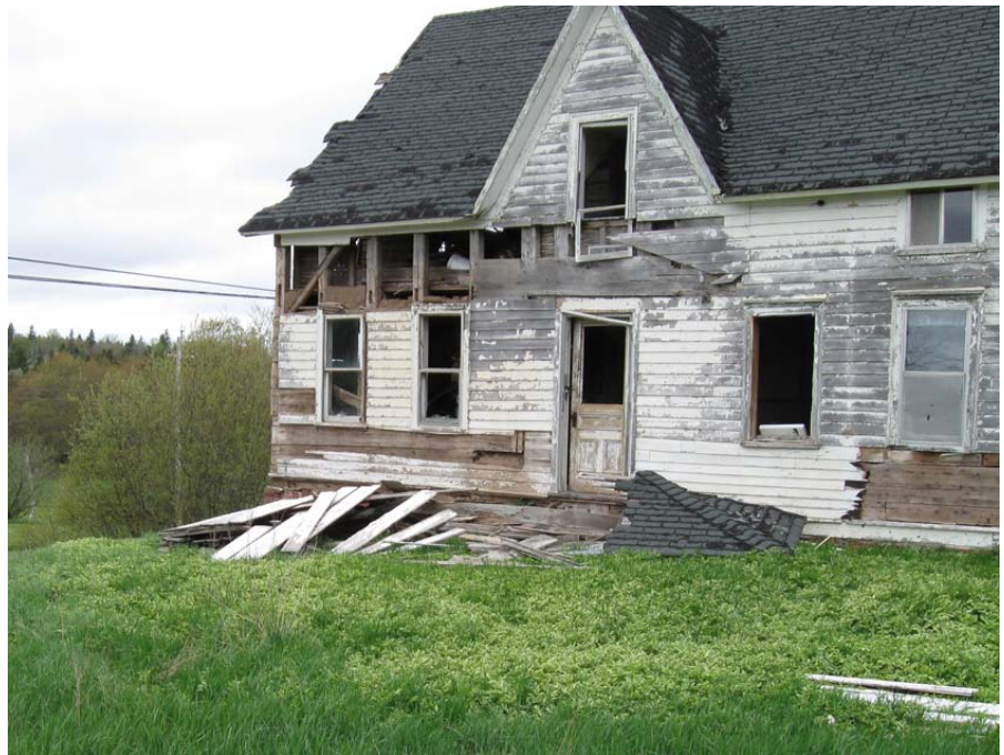
The home during demolition (all photos courtesy of the author)
