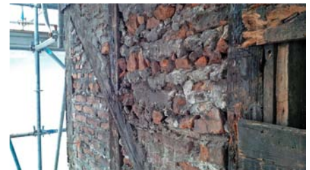
Timber frame structure with brick nogging (sheathing removed) (photo by Don Forbes)
