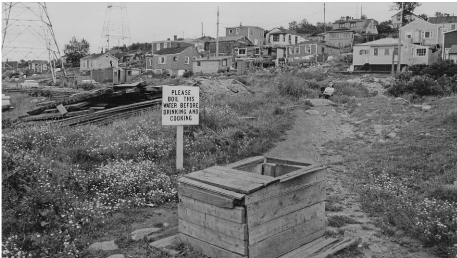
One of several wells that were the only sources of fresh water in Africville - the community did not receive the water and sewer services provided to other neighbourhoods in Halifax - photographer: Bob Brooks, black and white negative, contact print, ca. 1965 (courtesy of Nova Scotia Archives, accession no. 1989-468 vol. 16/ negative sheet 6, image 31)
