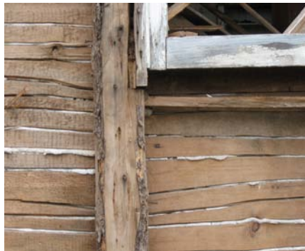
Plaster lathes were split, not sawn
