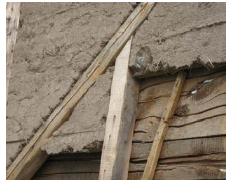
Walls were filled with a mud and straw mixture
