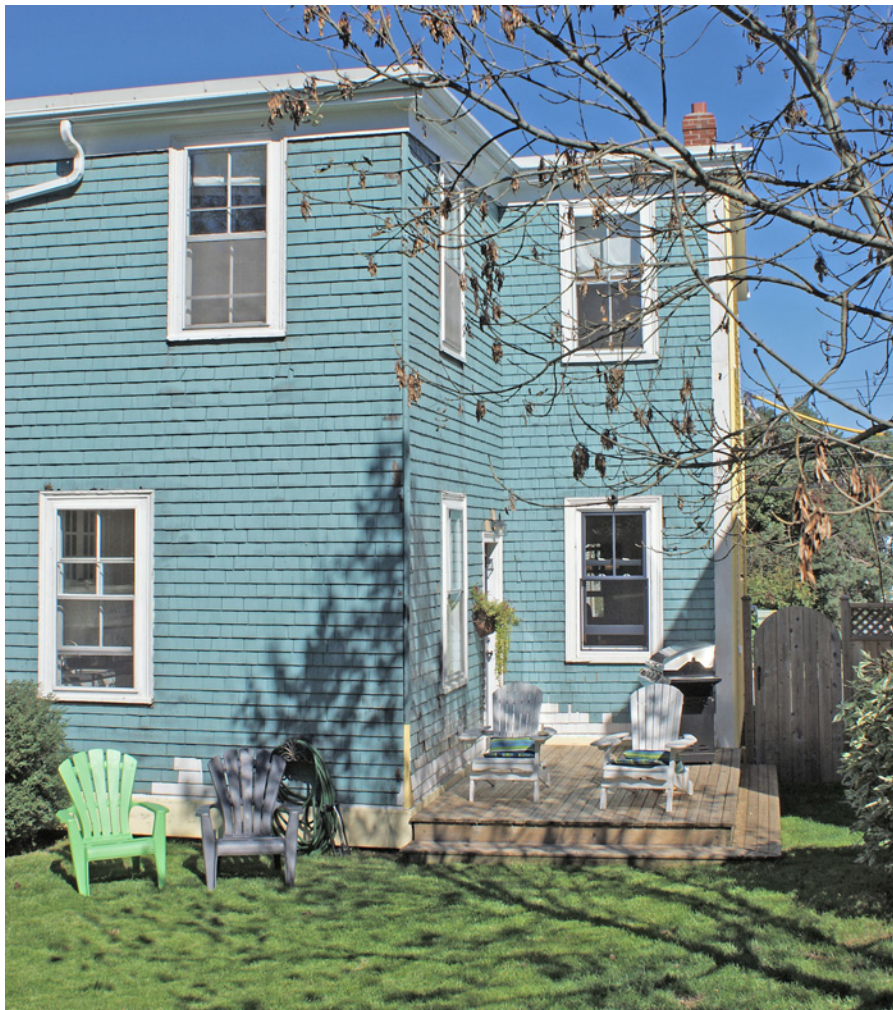
Rear view of 23 Pine Street in 2013 (courtesy of Hal Oare)
