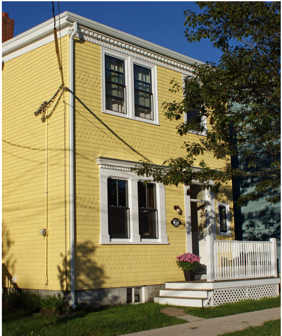
23 Pine Street in its restored finery, 2013 (courtesy of Hal Oare)
