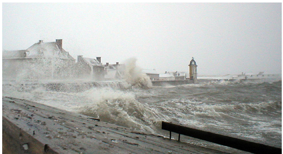
Waves overtopping the seawall at Louisbourg in a major storm (courtesy of Ian Harte, Parks Canada, with assistance from Bob Taylor, Geological Survey of Canada)
