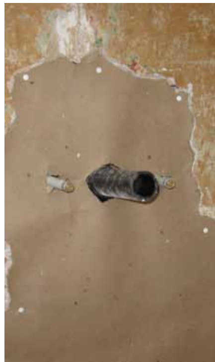
A paper template has been cut in place. Note the thumb tacks.
