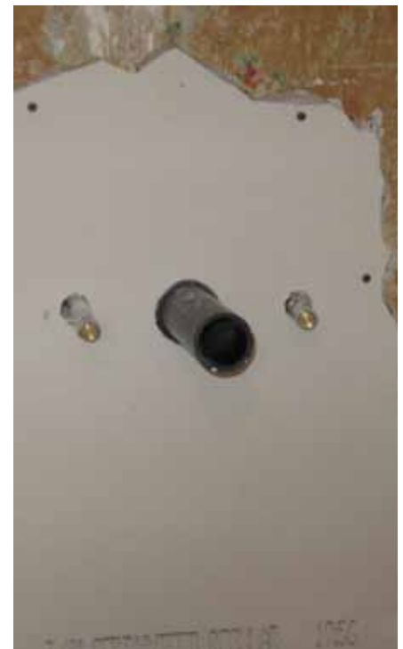
The damaged area patched with drywall prior to taping.
