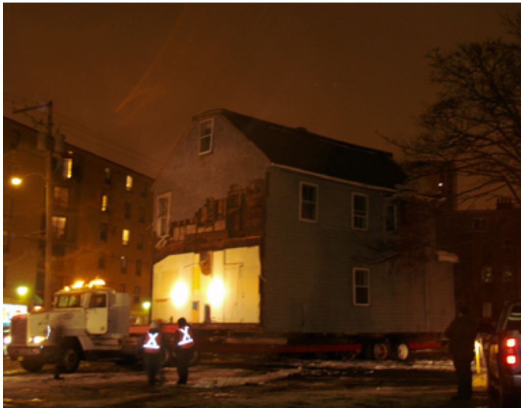
Night falls as the Morris house nears completion of its 2009 move onto the Nova Scotia Power property on Water Street where it rested for over three years. (Courtesy of Aaron Murnaghan)
