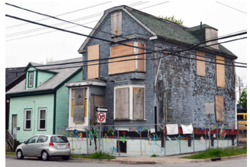
The house was parked at the back of the lot until the foundation was ready. Note heavy wires on both streets. Manoeuvring across the double bundle and onto the narrow lot was difficult. (Courtesy of Don Forbes)
