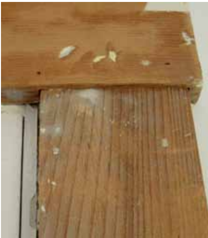
The side casing fits into a pocket on the under side of the head-trim. Notice the slight head-trim extension at right.
