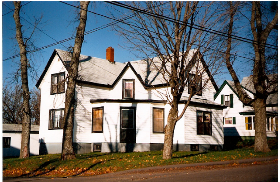
136 Main Street, Springhill, Nova Scotia. This cruciform house has ridgelines of matching height. (Courtesy of Springhill Heritage Group)
