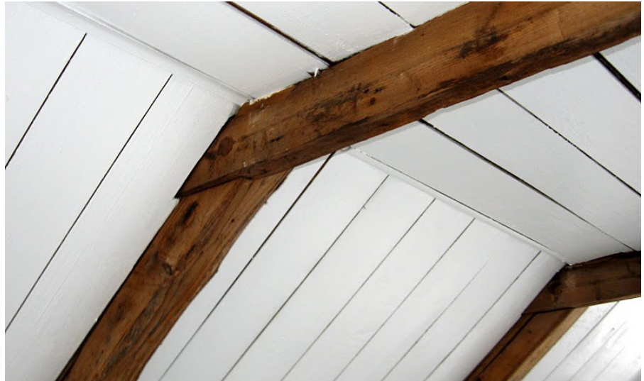
Exposed ceiling joists.
