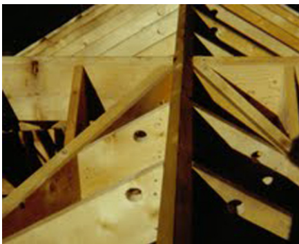
Two ridges and four valleys collide on this 4-gabled pool house framed by the author at West Tisbury, Massachusetts.
