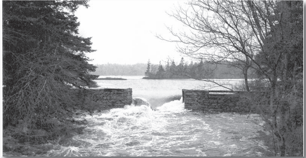
The dam as it looked at the beginning of the restoration.
