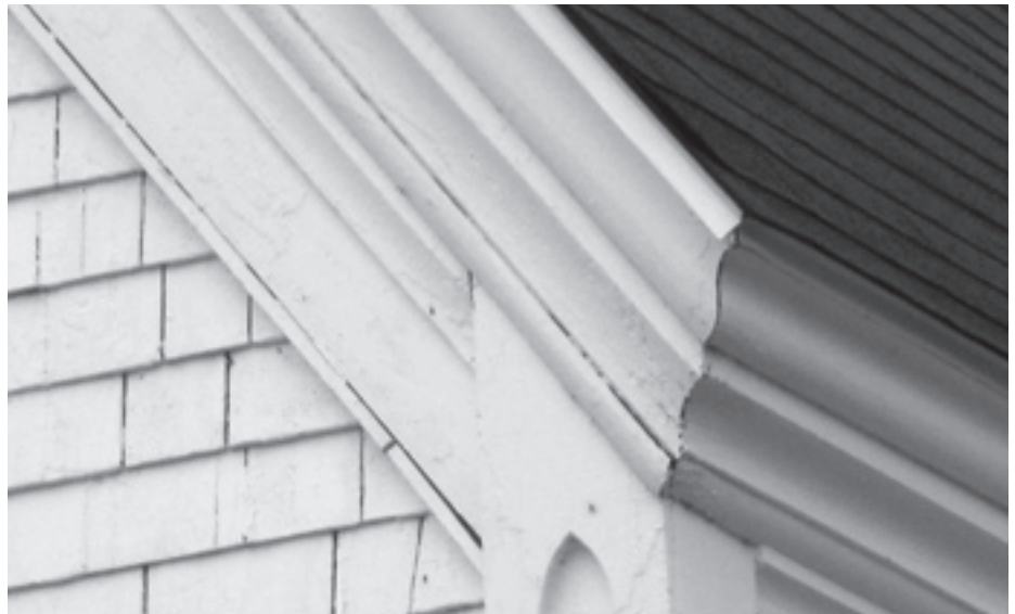
Photo 2: Where the level crown meets the gable crown is an impossible woodworking joint. Location: St. Mark's Church, Martin's Point, Nova Scotia. (Bruce MacNab)
