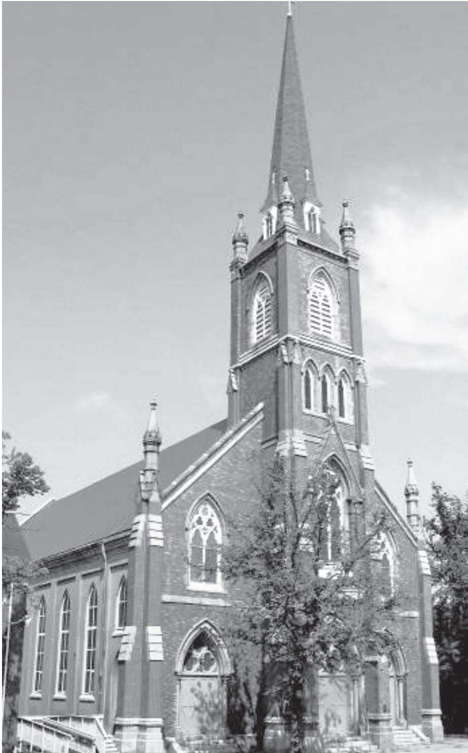
St. Patrick's Roman Catholic Church, Brunswick Street, Halifax, is Victorian Gothic in style. The brick construction is trimmed with Nova Scotia granite while the sides are faced with stucco. The symmetrical front façade has typical Gothic detailing: hood drip moulds, spires, window tracery and buttresses. The cornerstone was laid in 1883. (Photo by Arianne Pollet-Brannen)
