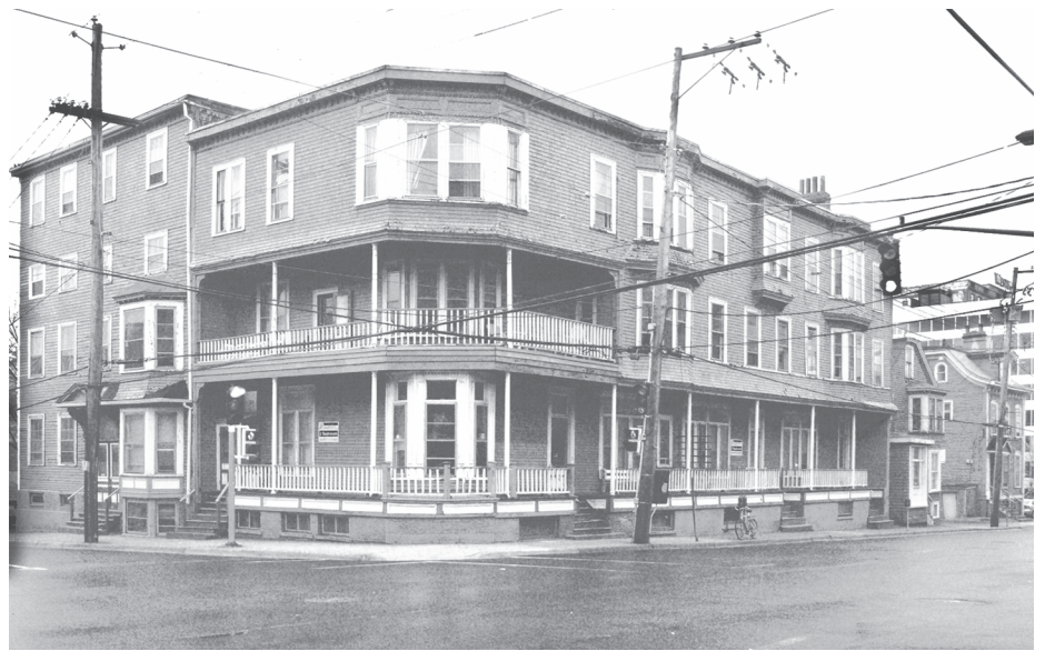
At the corner of Hollis and Morris Streets, Halifax, a clutch of four historic buildings, once known as the Morris mansion, the New Victoria Hotel, the Morris Office building, and Ruhland House awaited demolition this fall. Everyone in the city is said to have known someone who lived in "the hotel".
