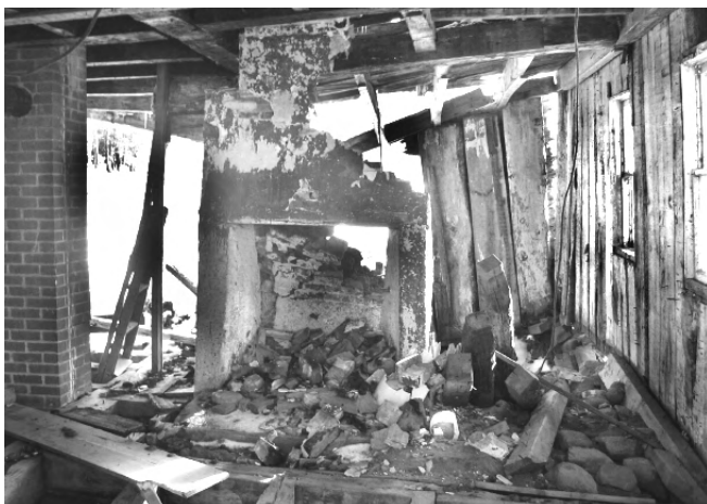
Construction details are exposed in 2009. (Peter Delefos)
