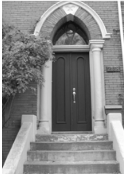
Below, 2138 Brunswick Street as part of the streetscape. Top left, the house, alone, and top right, its gothic revival entry.
