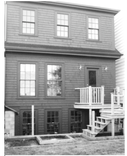
After (rear view)
