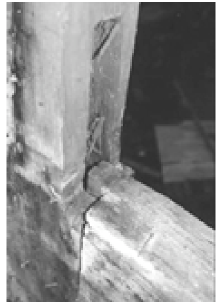
Detail of a wooden joint.
