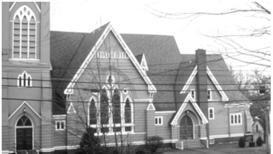
Saint John's Presbyterian Church and School House, King Street, now Windsor United Church.
