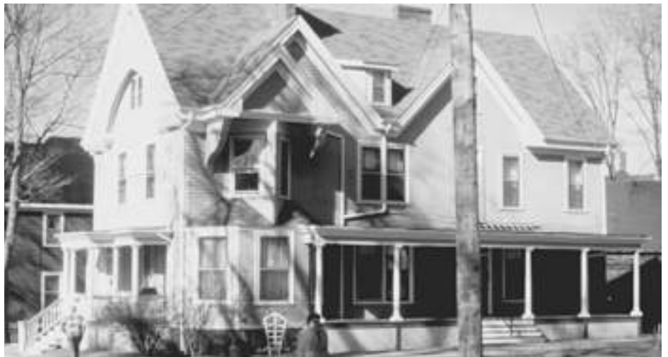
John C. Keith Residence, Clifton Street, 1898. This 2.5 storey home was 60x34 feet, with a back ell for cold storage 20x14 feet, a conservatory at the rear of the house, 24x24 feet. The interior was finished in Cyprus (sic), quartered oak and white wood. This house was also designed in the shingle or Stick style. At the same time a large barn, 42x24 feet containing stables, coach house, wood and root storage was built.
