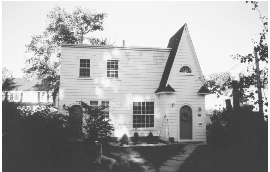
No. 981, the renovated coach house.
