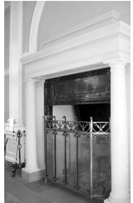
A truly spectacular example of a modified Rumford fireplace (the firebox is much larger than Rumford recommended) may be seen at the K. C. Irving Environmental Science Centre at Acadia University. Courtesy, Acadia University.
