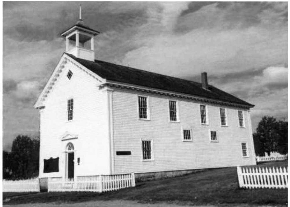
Argyle Township Court House (c.1803-05), Tusket, Yarmouth Co. It is the oldest surviving courthouse in Canada; the first court session was held here 29 October 1805. The building was restored in 1981-82. The ground floor contains the cell-block and jail-keeper's quarters; upstairs are the courtroom, grand jury room and the judge's chamber. At the rear on the ground floor is the Argyle Township Court House Archives, which contains all of the documents that survived in the building, many from the 1700s. Courtesy of Argyle Township Court House Archives.
