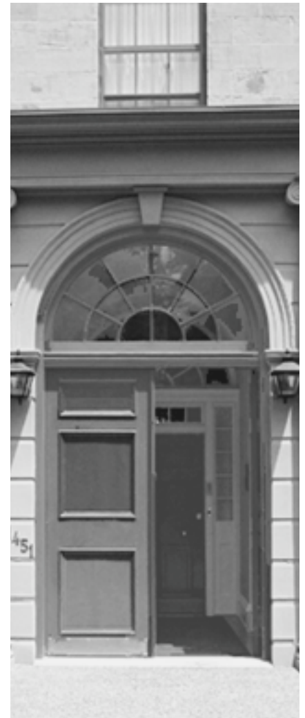
The Barrington Street entrance to Government House, the official Halifax residence of the Lieutenant Governor of Nova Scotia.
